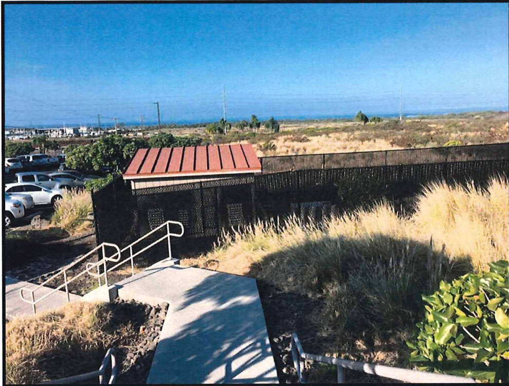
Kaiser Permanente Wastewater Treatment – Exterior View
