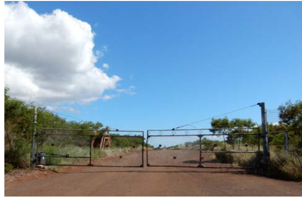
Photo 3. South gate off Akahahele Road.
