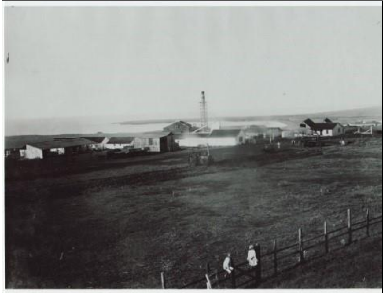
Figure 18. Photograph of sugar mill in 'Ele'ele, ca. 1885 (Post Office in Paradise 2015)
