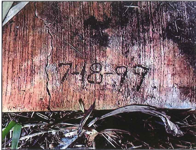
Figure 102. Photo of date discovered on the concrete floor of the abandoned shed, southeast of Site 73
