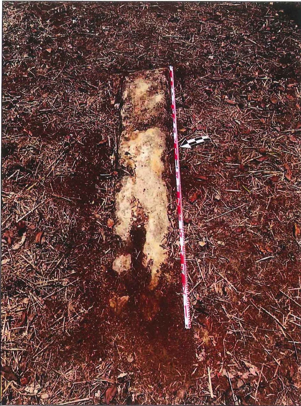
Figure 93. Photo of SIHP # -1501 Feature E-6, concrete slab embedded in road Feature C-3 on Aepoekolu dam, view to east
