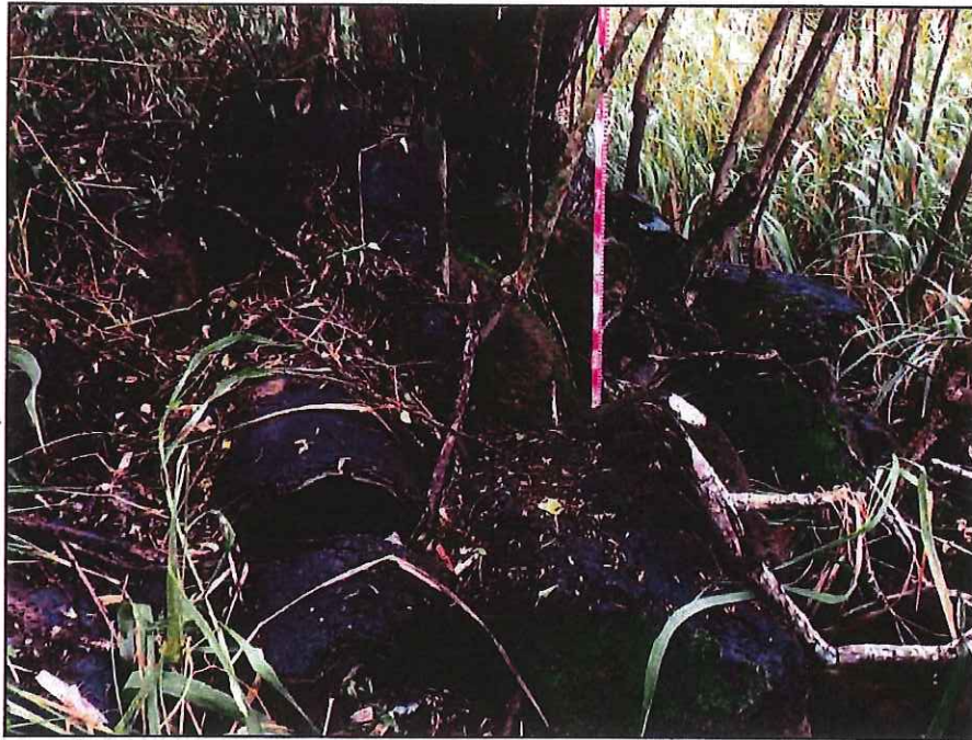
Figure 112. Photo of broken concrete pipe on the east portion of the push pile (Feature 0073-1), view to northeast
