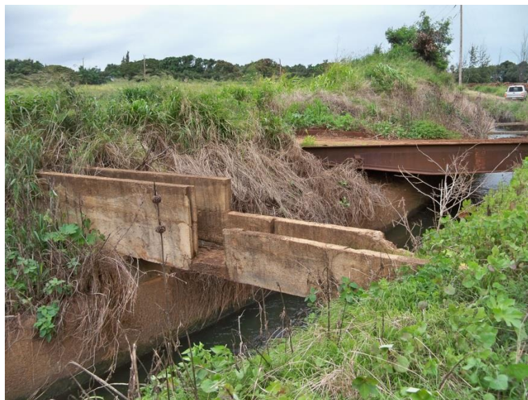
Figure 167. Overview Photograph of Second Bridge from the North, Metal Beam and Cement Construction (background), Older Drainage Culvert (foreground), View to Northeast
