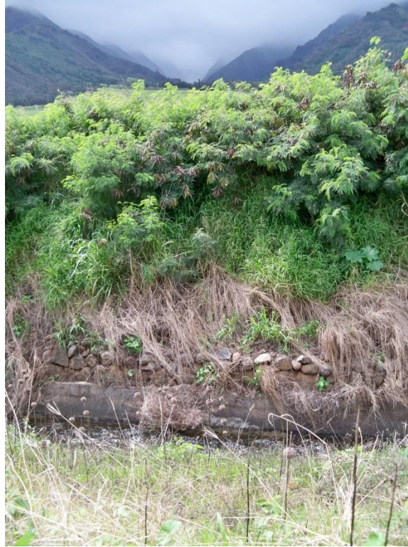
Figure 166. Overview Photograph of Site 5197 Waihe'e Ditch Showing Older Construction with Stacked Rock Atop the Concrete Lined Ditch (View of Western Side Wall
