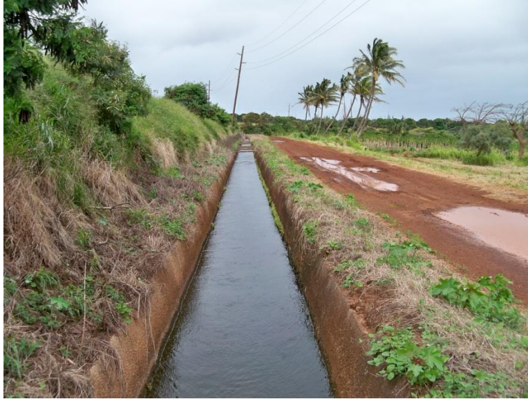
Figure 173. Overview Photograph of Site 5197 Waihe'e Ditch with Modern Concrete Lining, View to Northeast
