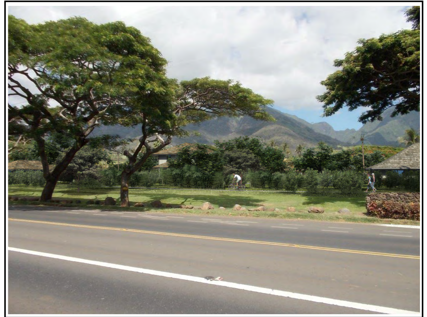
4. After. Looking in a south-westerly direction through the project with the West Maui Mountains in the background and the separated pedestrian and bicycle path in the foreground.
