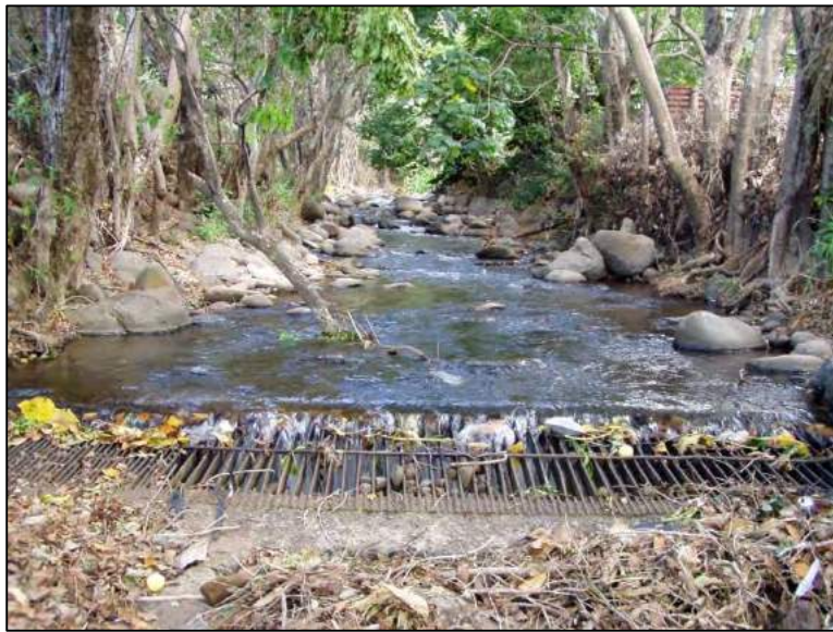
Figure 18. Lowest Waikapū Stream diversion located along Honoapiʻilani Highway in 2012 (Hökūao Pellegrino)
