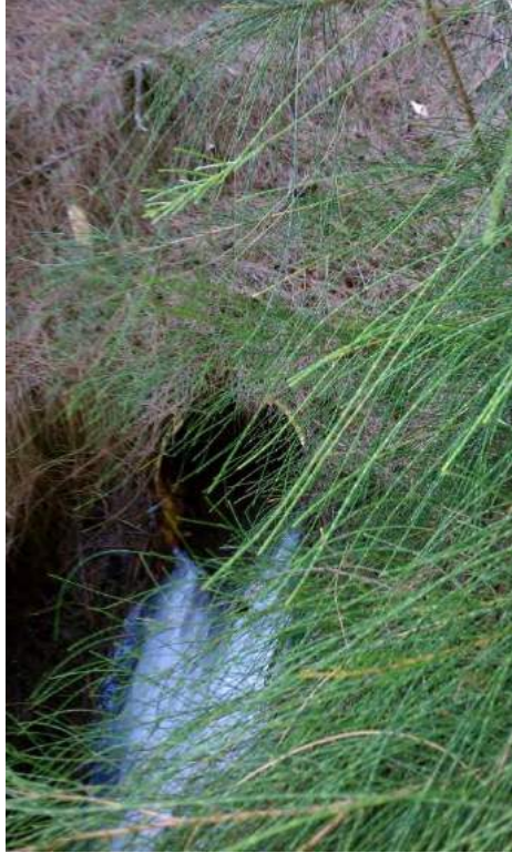
Figure 46. Photograph of Site 7881 Feature 11 Out-take (View to West)
