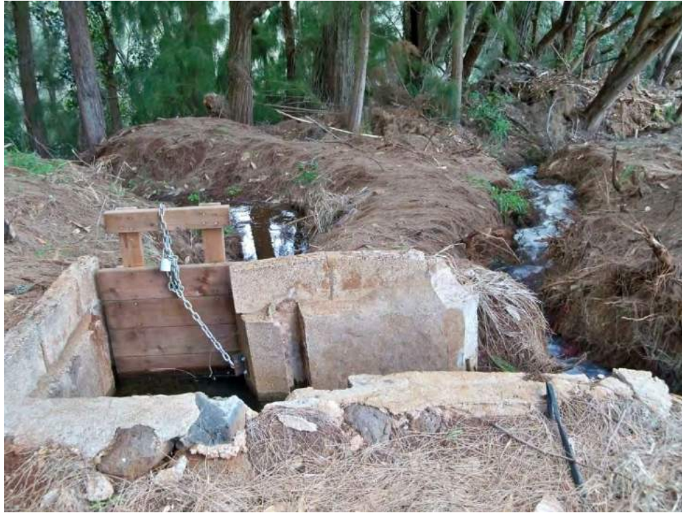
Figure 38. Photograph of Site 7881 Feature 8 showing Two Channels, Feature 2 Ditch continues East and Overflow beyond Sluice Gate to Waikapū Stream (View to North)
