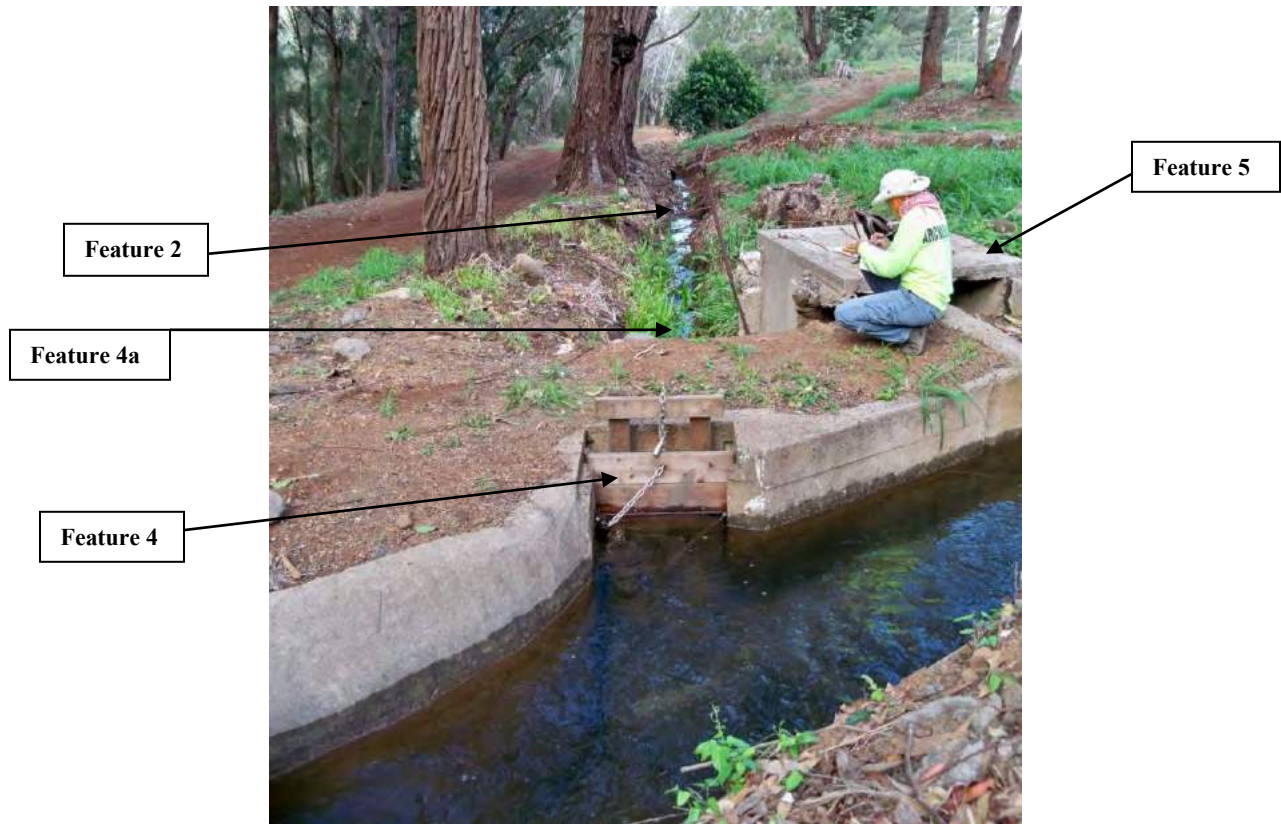
Figure 31. Photograph of Site 7881 Features 1 and 2 ditches and diversion structures Features 4, 4a and 5 (View to South)
