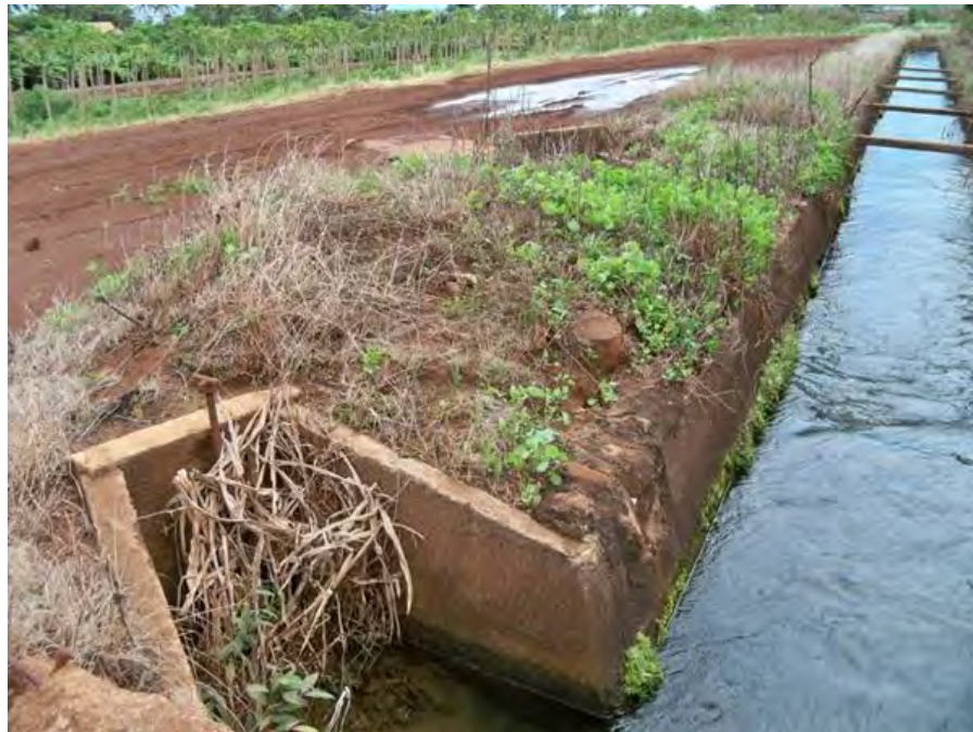
Figure 171. Overview Photograph of Third Bridge with Older Penstock with Metal Shut-off Valve (left), View to South
