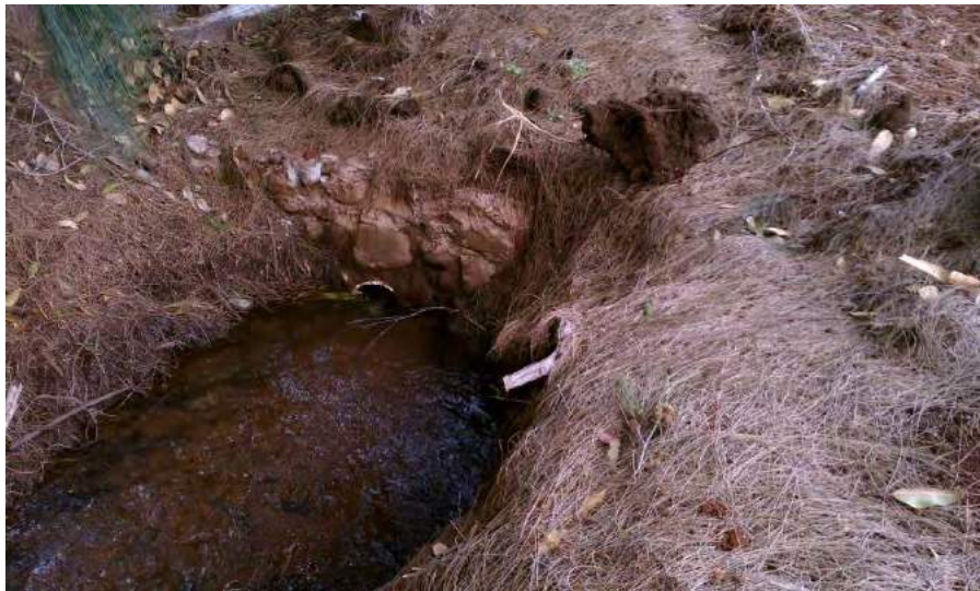
Figure 40. Photograph of Site 7881 Feature 9 Intake on West side (View to East)
