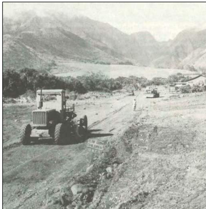
Figure 26. Preparing Waikapū Subdivision for house lots in 1955 (W.S.Co)
