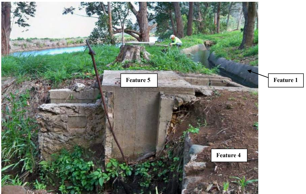
Figure 32. Photograph of Site 7881 Features 4, 4a and 5 Water Diversion Features (Bottom)
