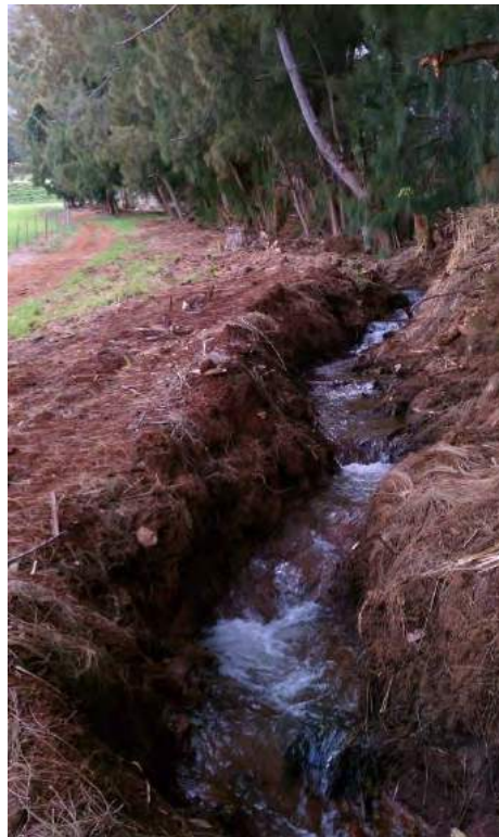
Figure 44. Feature 2 Ditch flowing into Site 7881 Feature 10 Culvert (View to West)
