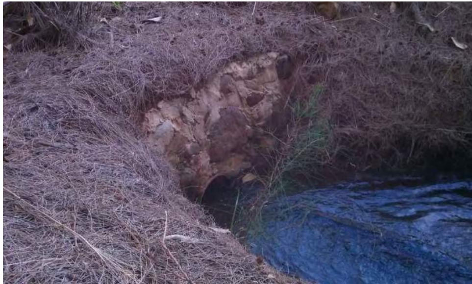
Figure 45. Photograph of Site 7881 Feature 11 Intake on West (View to East)
