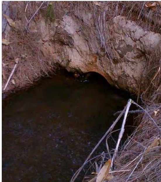
Figure 42. Photograph of Site 7881 Feature 10 Intake on West (View to East)
