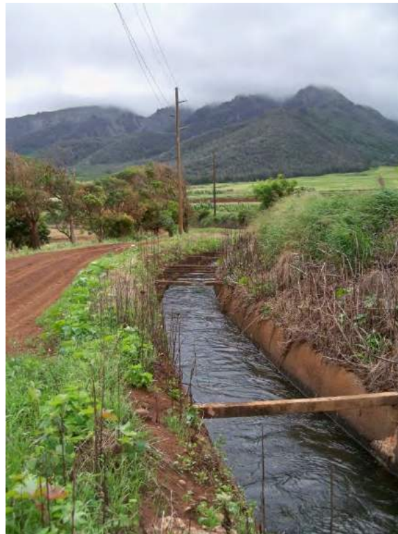
Figure 169. Photographic Overview from Second Bridge with Tee-Bar Reinforcements Across Ditch, View to Southwest
