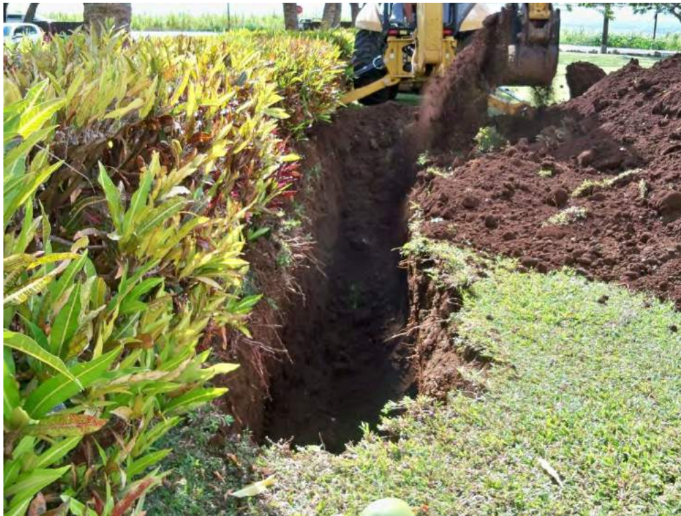
Figure 152. Overview Photograph of Trench 318 Base of Excavation
