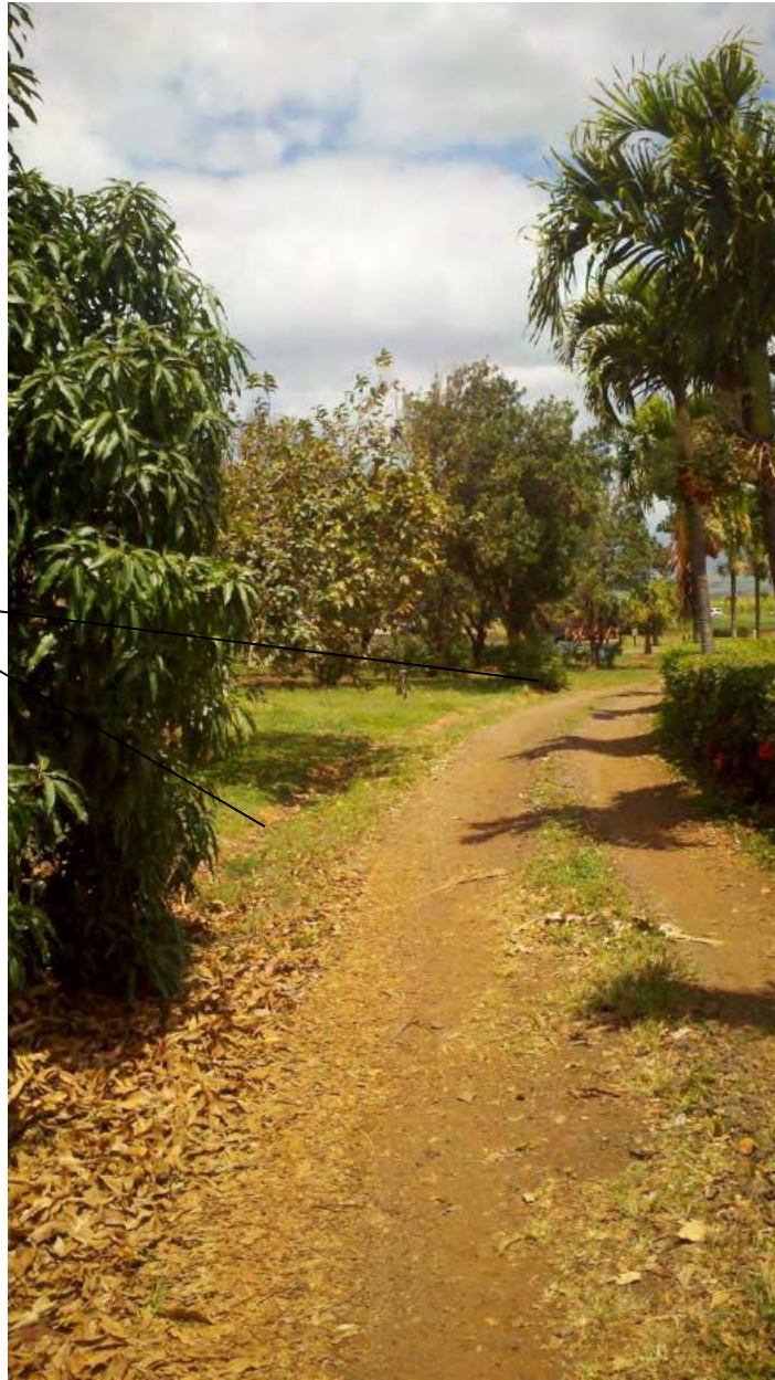
Figure 175. Overview Photograph of Concrete Swale along Cane Flume Easement
