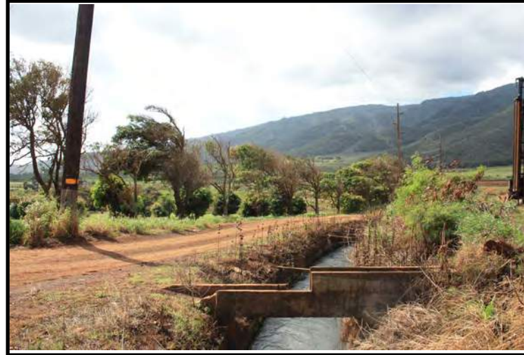
32. Looking southwest at the existing Waihe`e irrigation ditch that lies north to south across the property.
