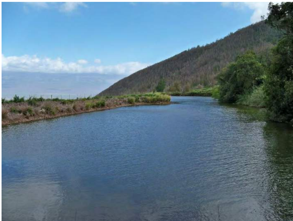
Figure 29. Site 7881 Feature 3 Reservoir, View to South
