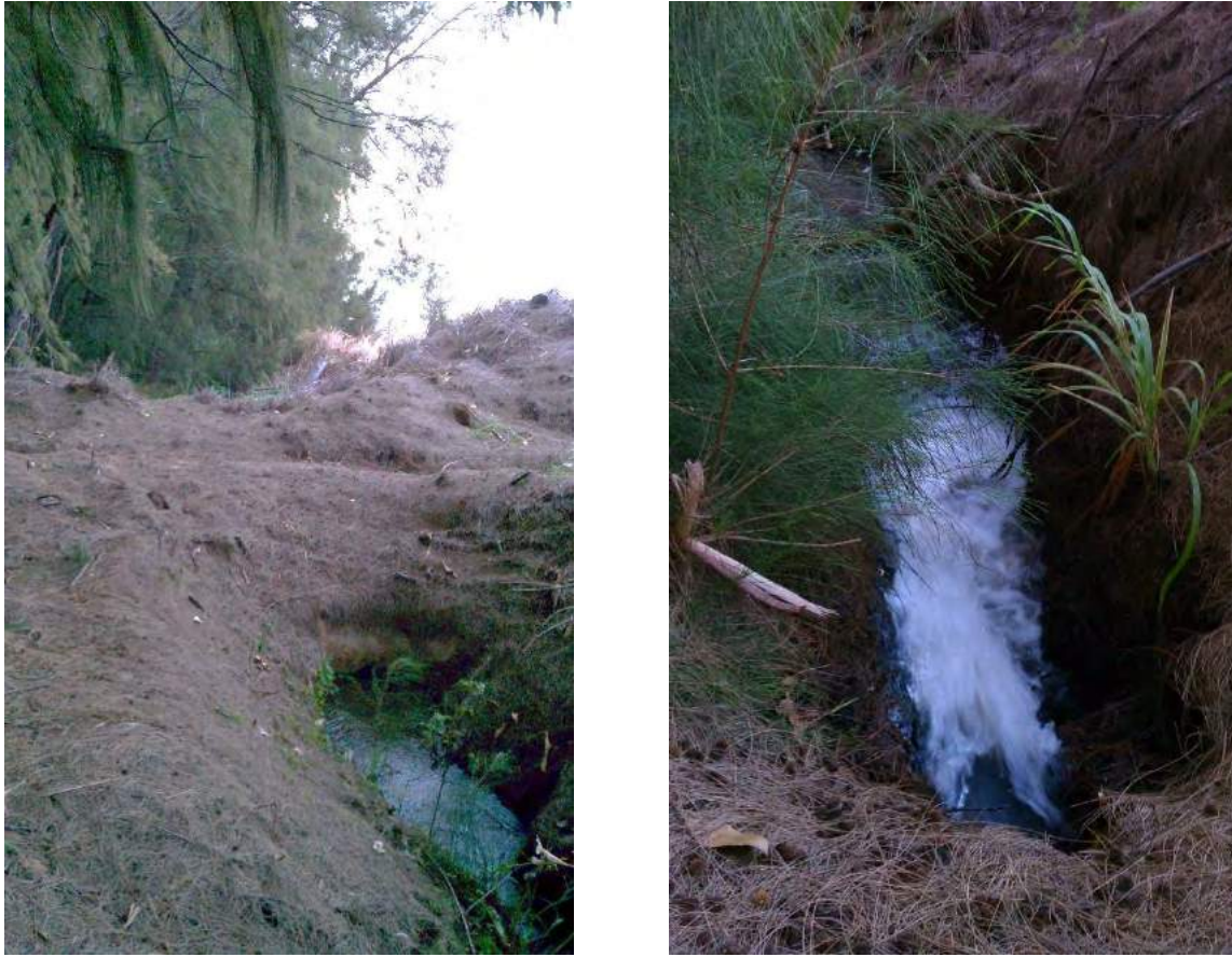
Figure 48. Photographs of Site 7881 Feature 13 Intake (View to East) left; Feature 13 Out-take (View to West) right
