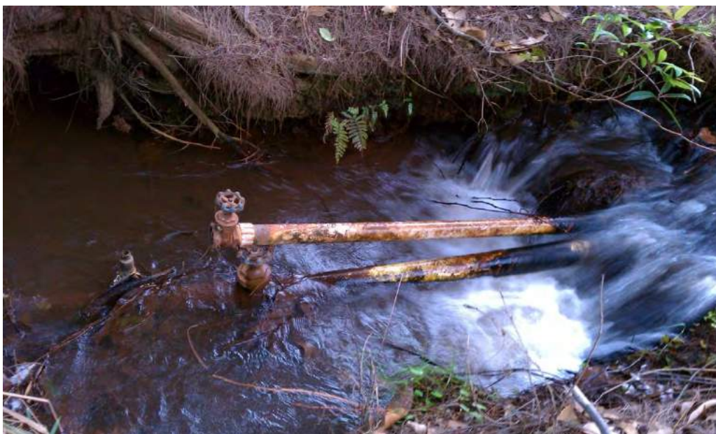
Figure 54. Photograph of Site 7881 Feature 17 Valves (View to South)
