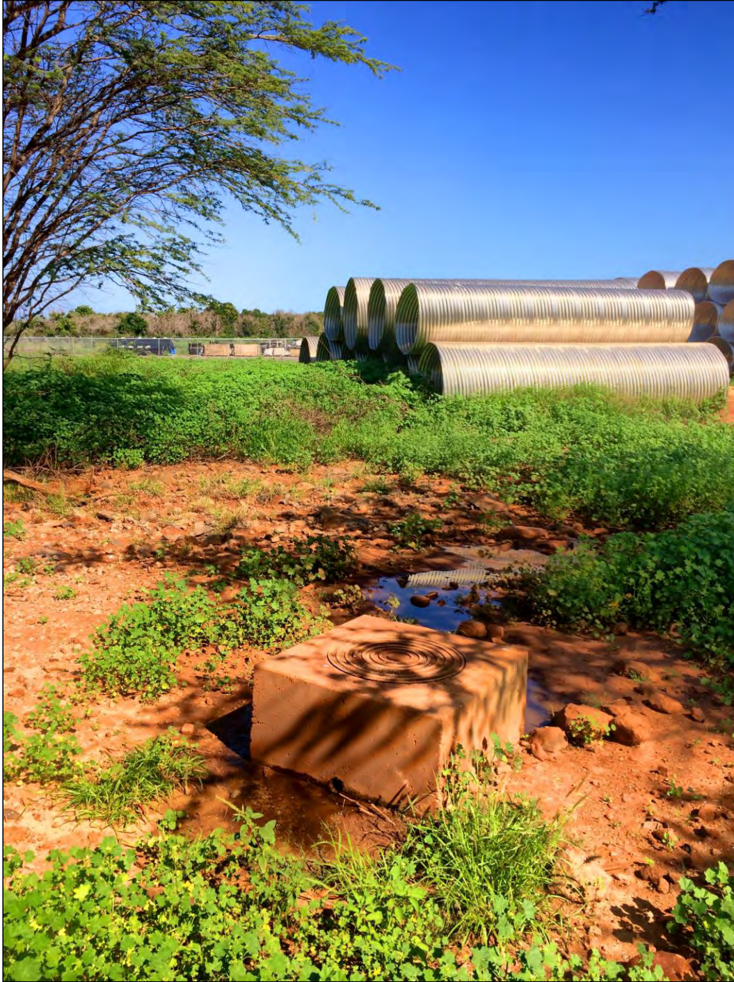
Photo 5: Photo showing the existing waterline manhole near the northeast of the base yard. This water line will be abandoned and a new waterline will be installed along the east and south border of the Piilani Promenade project area.
