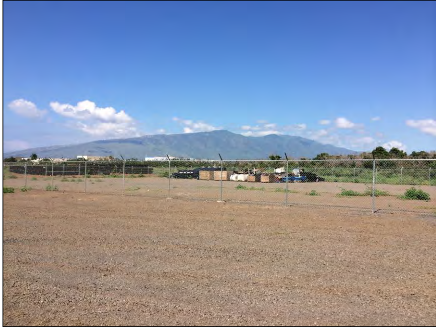
Photo 8: Base yard on portion of Piilani Promenade. Note the fenced area is owned by Honua`ula Partners, LLC. View to the northeast.
