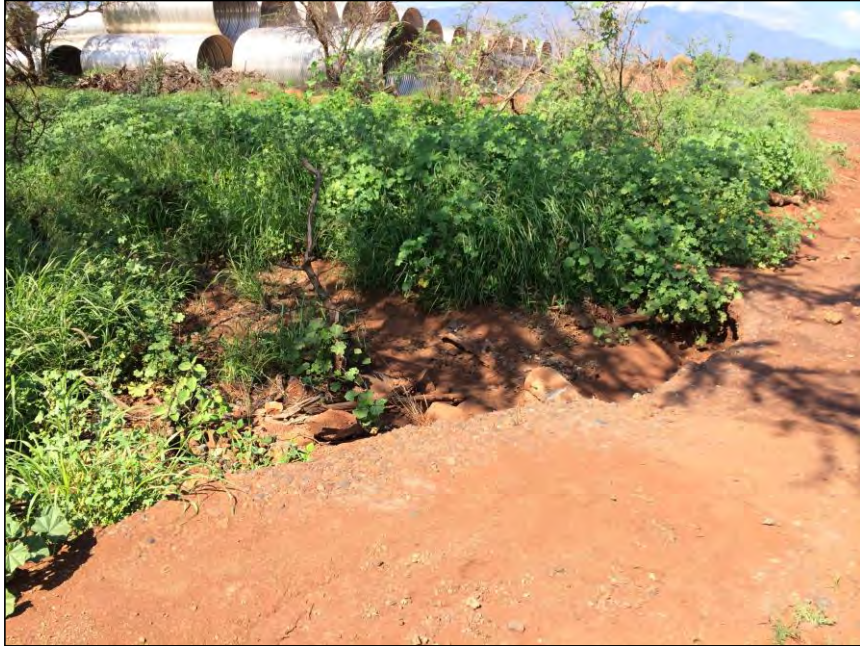
Photo 6: Small drainage gully that crosses Lot 2B near the base yard.
