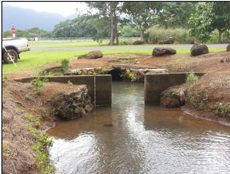
Figure 84. Photo of SIHP # -2179 Feature A3, sluice gate at the southwest side of the Feature A overflow area, view to south
