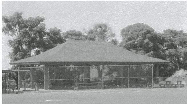
Pavilion at Kaumakani Park
