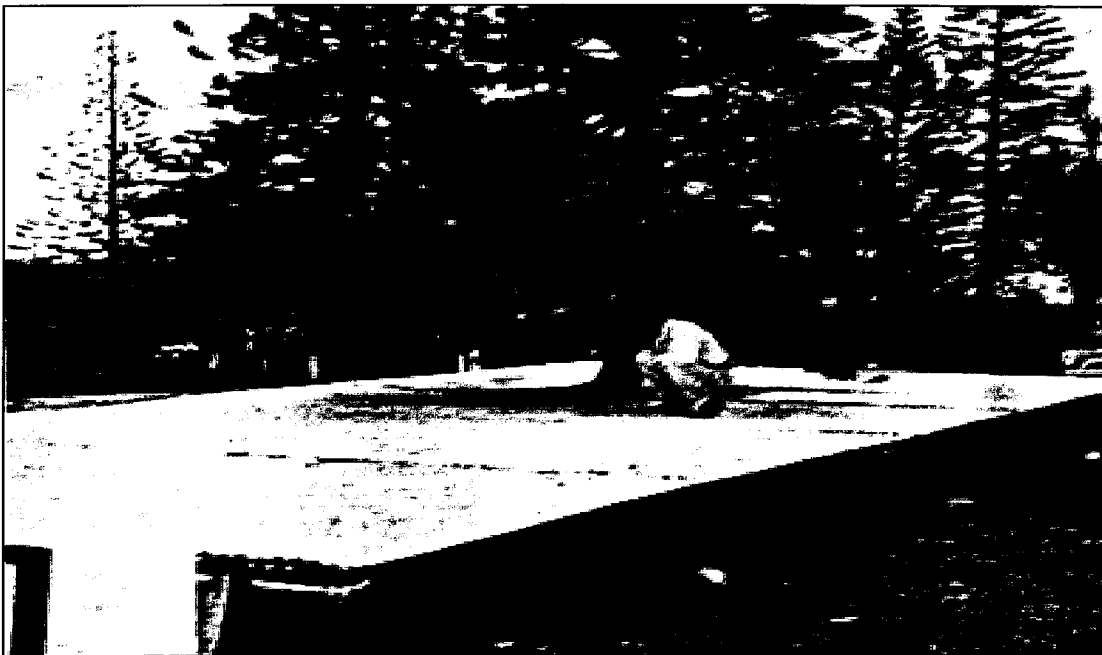
Figure 7. Full canopy sheet-metal catchment installed under Cook pine during 1950s PRI study.
