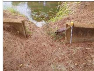
Figure 17. CSH 1, abandoned irrigation ditch, showing the reservoir adjacent to and northeast of the project area and a concrete gate frame that lacks a gate, view to west
