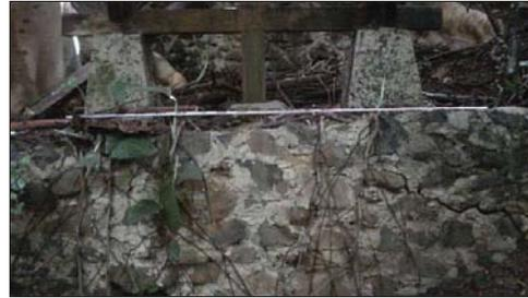
Figure 36. CSH 8, flume, showing concrete and boulder retaining wall beneath flume, view to east
