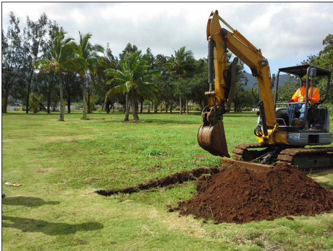
Figure 64. General location of T-9, view to south
