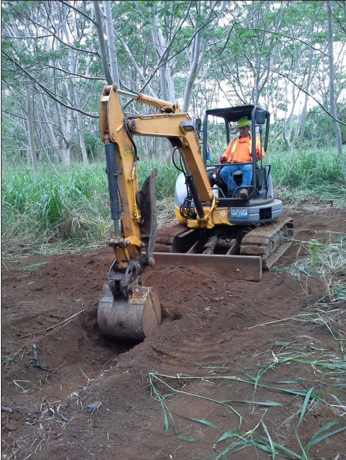
Figure 58. General location of T-7, view to south
