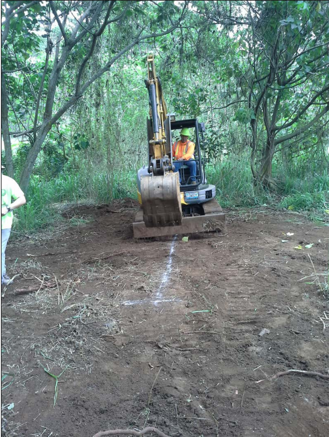
Figure 52. General location of T-5, view to east
