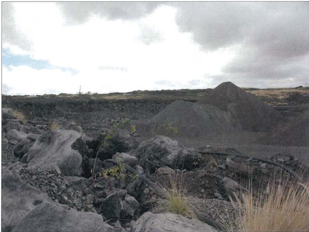
Figure 7. Quarrying activity within the central portion of the study area, view to the northeast.
