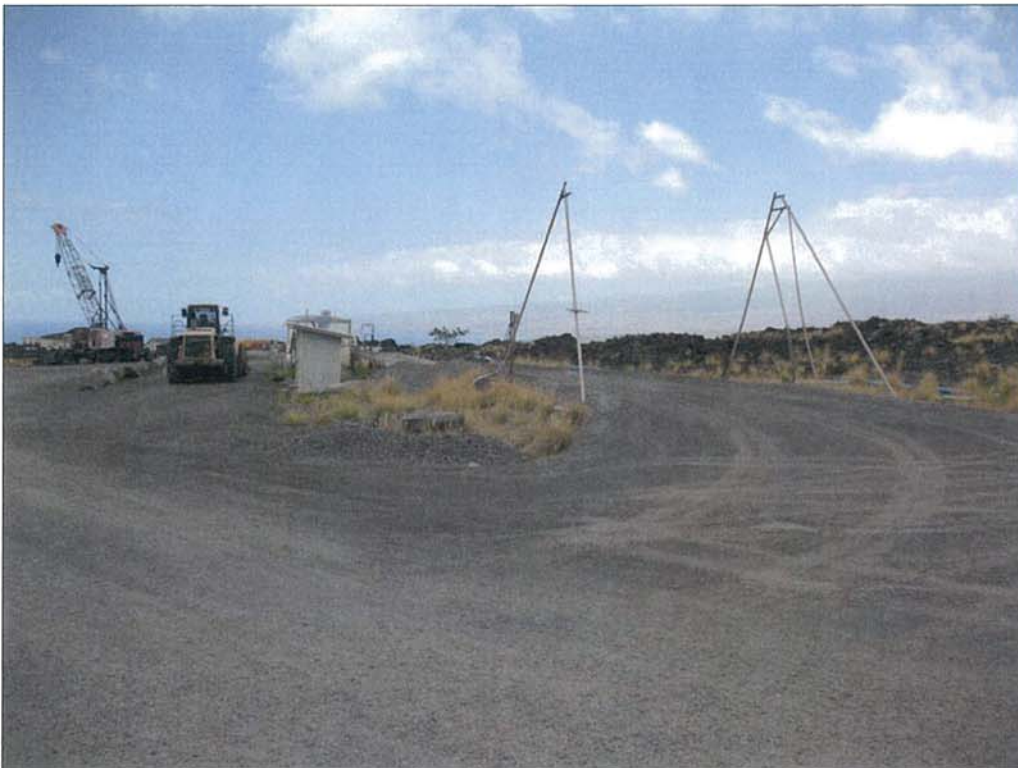
Figure 5. Weigh station and graded access road near the entrance to study area, view to the northwest.
