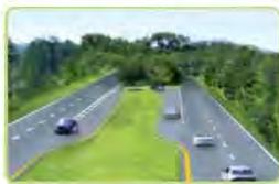
The Olowalu O-turn keeps traffic flowing continuously without stoplights or over/underpasses. The design features long merge lanes which allow for easy turns.
