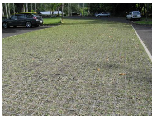
Figure 3-2. An application of permeable paving
