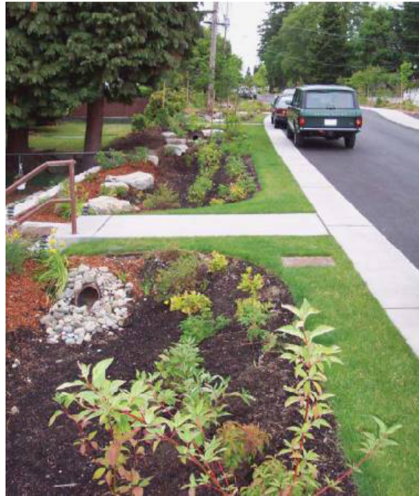
Figure 2-1. A bio-retention rain garden
