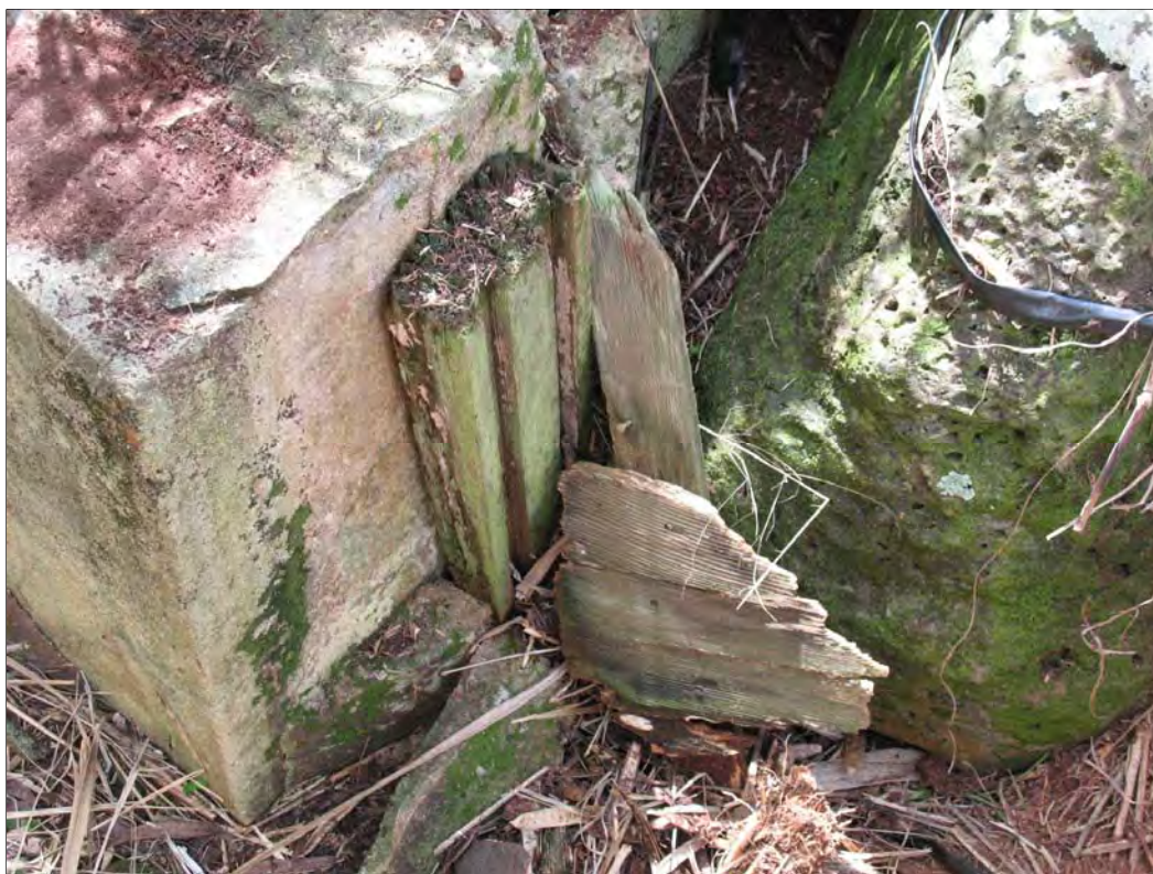
Figure 69. Site 7712 example of double wooden sluice gates controlling water flow into adjacent fields, view to the southwest.
