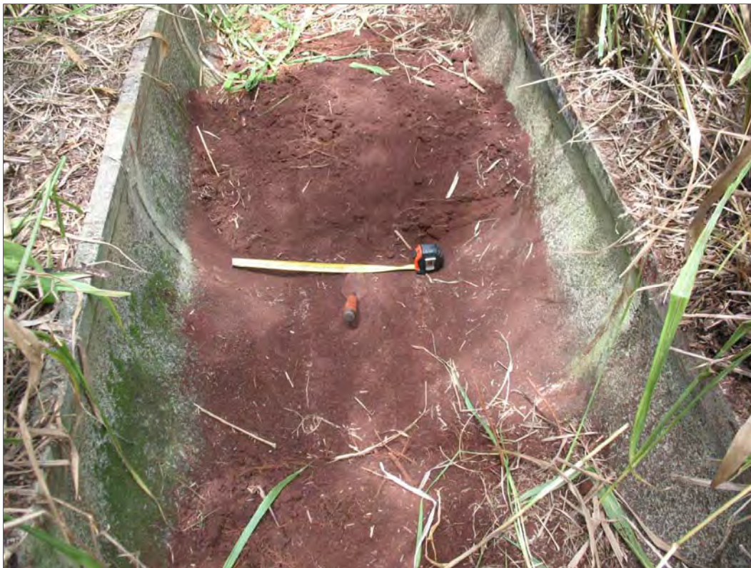
Figure 67. Site 7712 showing sectional concrete ditch elements.
