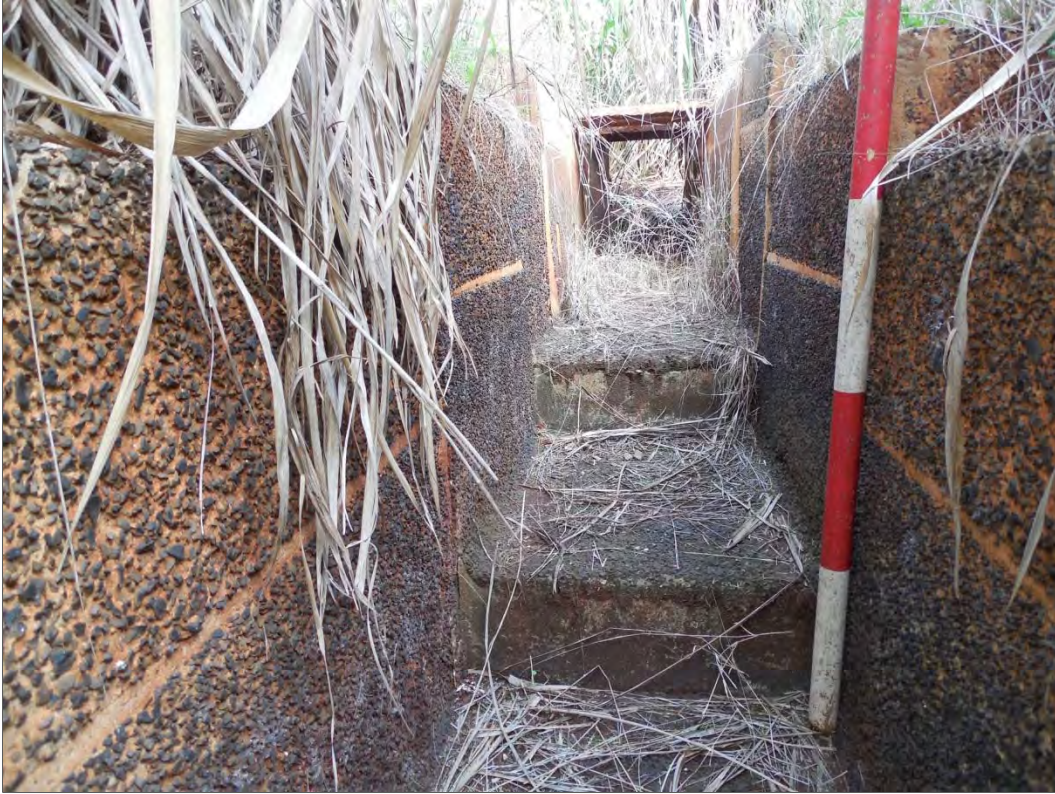
Figure 61. Site 7171, stepped concrete channel between the ditch and the southern end of the makai retention pond, view to the east.
