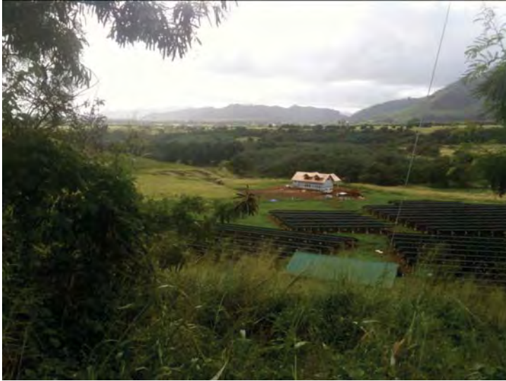
Figure 9. KIUC's Solar Farm and Equipment Buildings.
