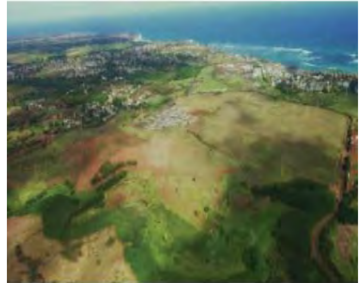
Figure 2. Aerial View of Project Area Looking North
