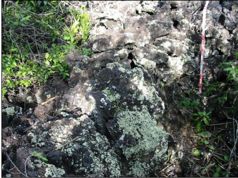
Figure 106. SIHP # 50-10-28-26436, Feature A, photograph of informal wall across natural depression
