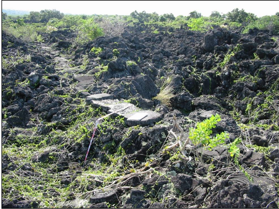
Figure 45. SIHP # 50-10-28-26418, photograph of Section D, showing partially constructed causeway along trail
