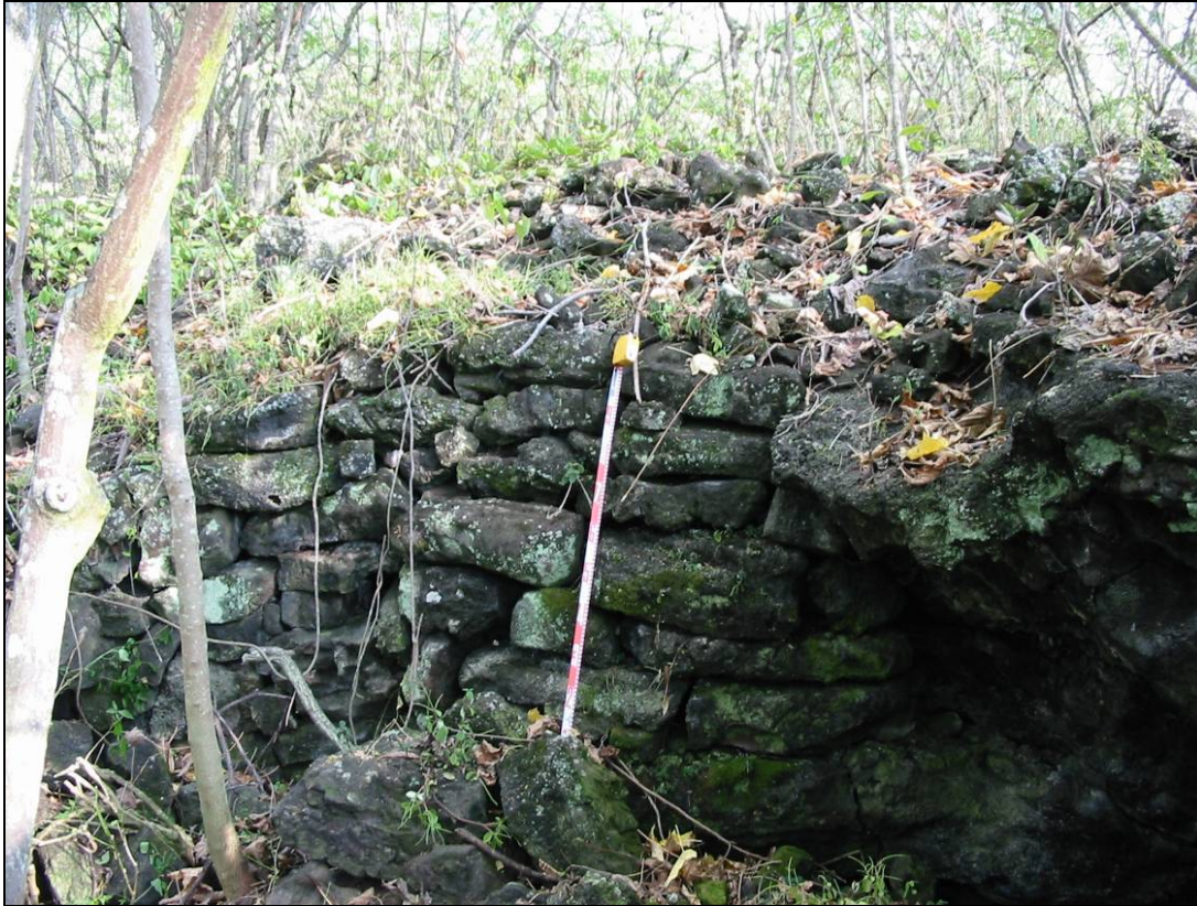
Figure 118. SIHP # 50-10-28-26440, Feature A, photograph of retaining wall facing east
