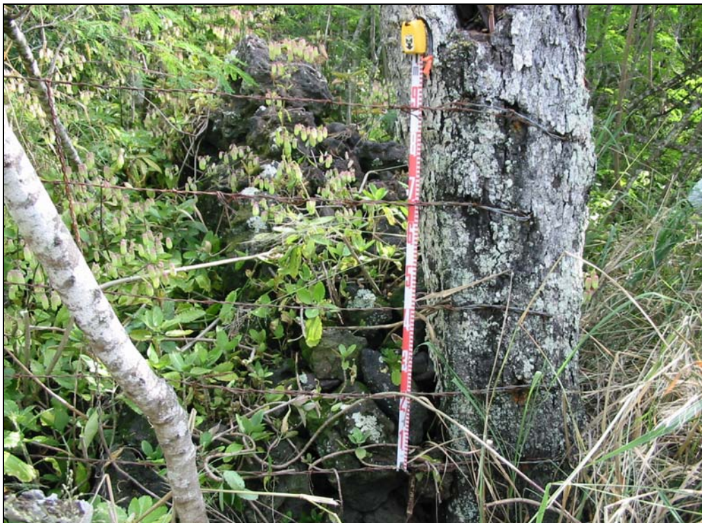
Figure 145. SIHP # 50-10-28-26450, photograph of wall where it abuts barbed wire fence
