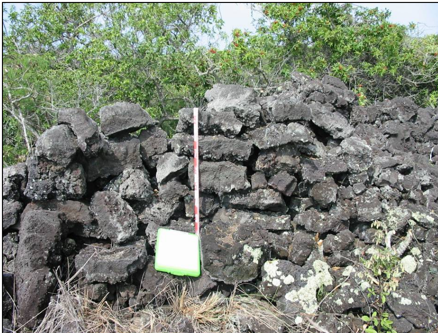
Figure 128. SIHP # 50-10-28-26443, photograph of southwest corner facing north, showing Area 3 (standing in Area 4)
