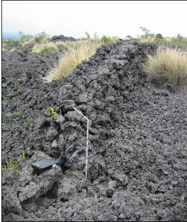
Figure 19. SIHP #50-10-27-26414, photograph looking southeast at 'a 'ā portion of historic wall
