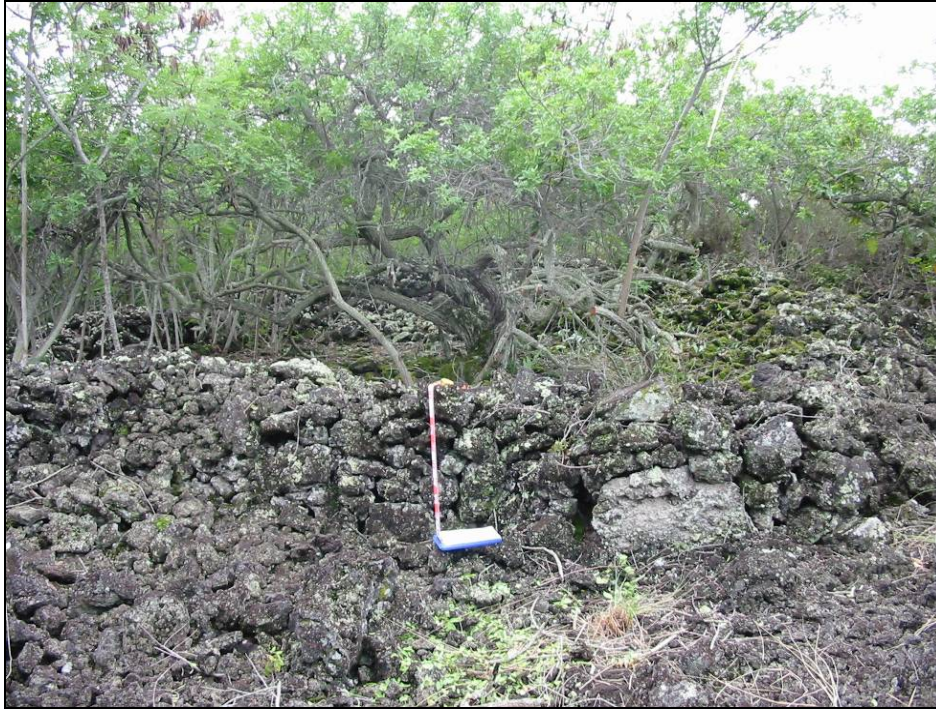
Figure 57. SIHP # 50-10-28-26424, overview photograph of enclosure facing southeast, north wall in foreground
