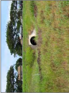
Photo 19 Stormwater Culvert Located Adjacent to Western Property Boundary on Pʻiliani Highway
