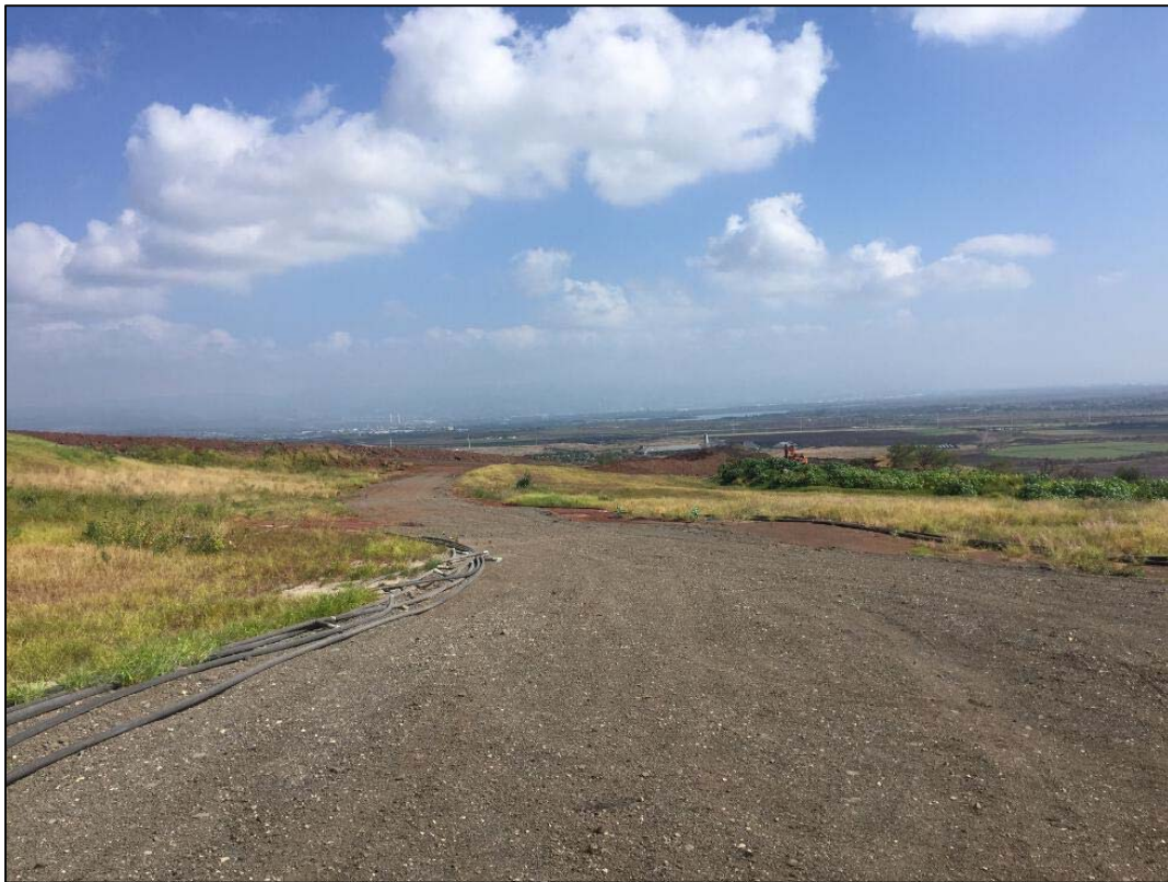
Photo 14. Recycled asphalt placed on access road near Hole 9 to reduce dust, facing east.
