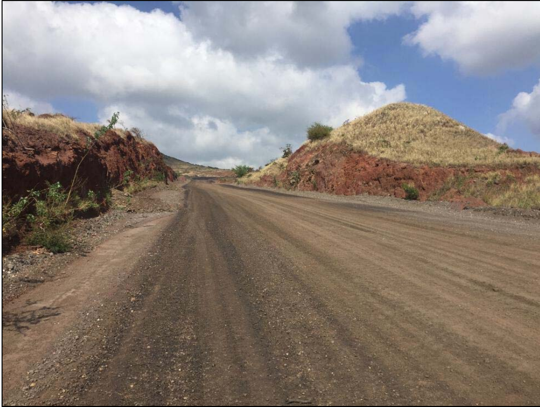
Photo 13. Recycled asphalt placed on west haul road to reduce dust, facing mauka.
