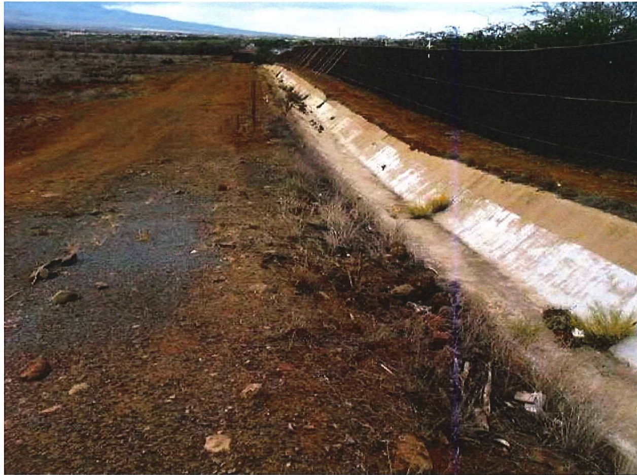
View of concrete drainage culvert that runs along the western boundary of the subject property and under Piilani Highway.
