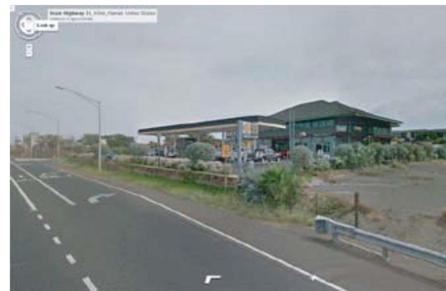
Blackie's Pit Stop (center) - northeasterly view
