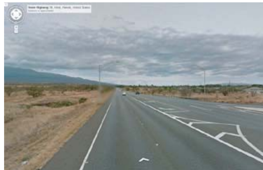
Project Site (left) and Pi'ilani Hwy (right) - southerly view
