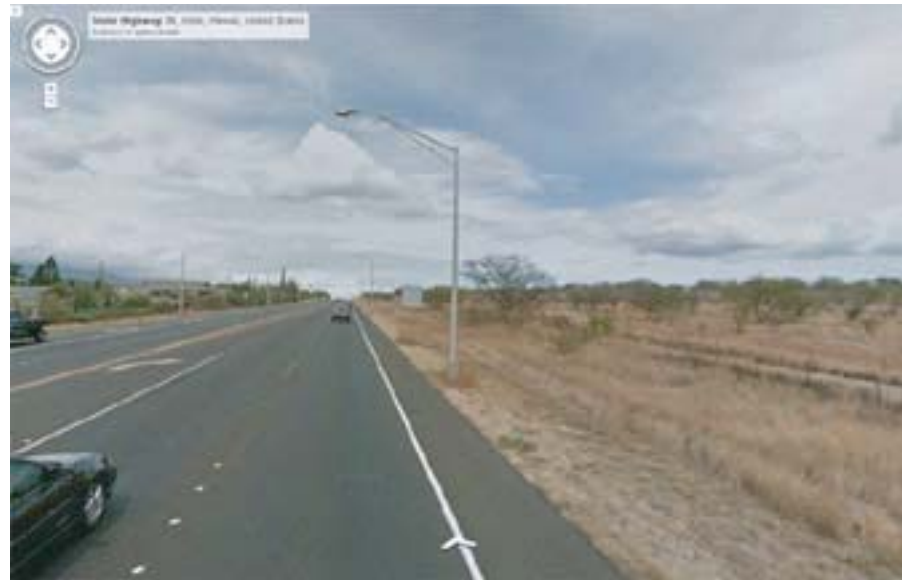
Pi'ilani Hwy (left) and Project Site (right) - northerly view
