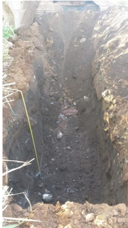
Figure 29. Overview Photograph of Trench 8 (View to East)
