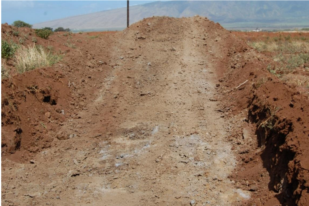
Figure 23. Overview Photograph of Bulldozer Cut 2 (View to West)
