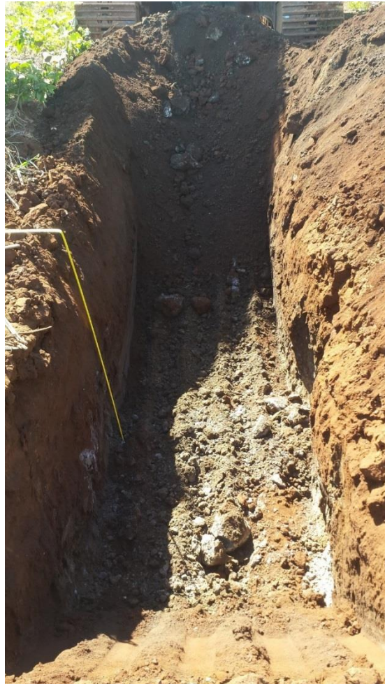
Figure 33. Overview Photograph of Trench 10 (View to East)
