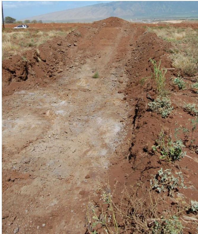
Figure 21. Overview Photograph of Bulldozer Cut 1 (View to West)
