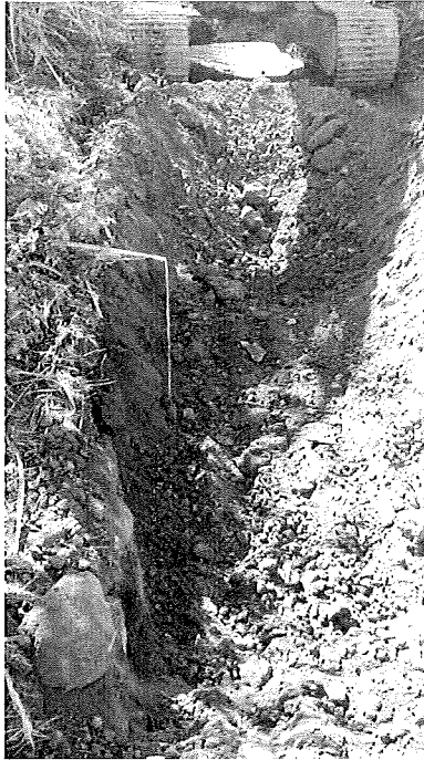
Figure 31. Overview Photograph of Trench 9 (View to East)
