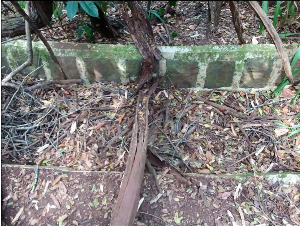
Photo 11. Example of a concrete and stone lined ditch found within the Study Area; December 2020.
