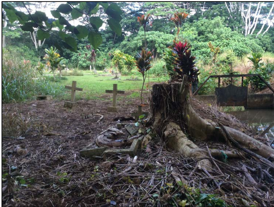
Figure 243. Feature M3, sluice gate, showing close proximity to SIHP # -B006, view to northeast
