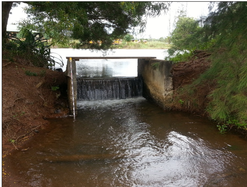
Figure 106. Photo of SIHP # -2179 Feature A1, sluice gate at the northern end of the overflow area, view to north (Hunkin et al. 2014)
