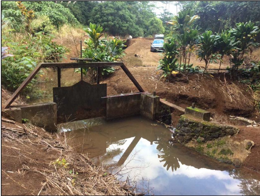
Figure 244. Sub-feature M3 showing north gate (left) and east gate (right), view to northeast
