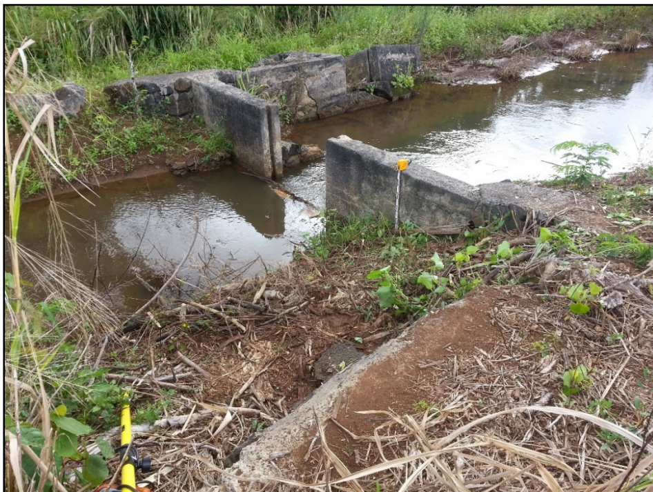
Figure 135. Photo of SIHP # -2179 Feature C2, view to southeast (Hunkin et al. 2014)
