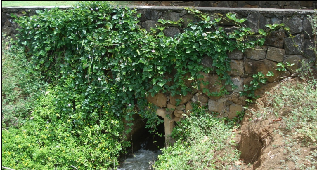
Figure 200. Sub-feature I3, view of concrete-lined culvert for Feature I, view to north
