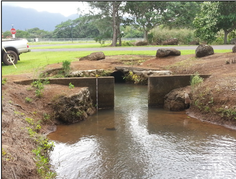
Figure 110. Photo of SIHP # -2179 Feature A3, sluice gate at the southwest side of the Feature A overflow area, view to south (Hunkin et al. 2014)
