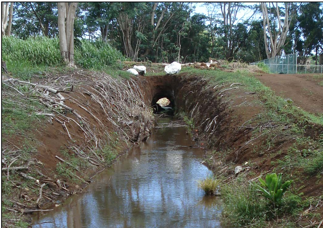
Figure 250. View of tunnel and roadway associated with Sub-feature M4, view to north
