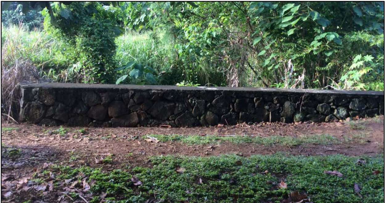
Figure 199. Sub-feature I3, retaining wall of culvert on south end, view to south
