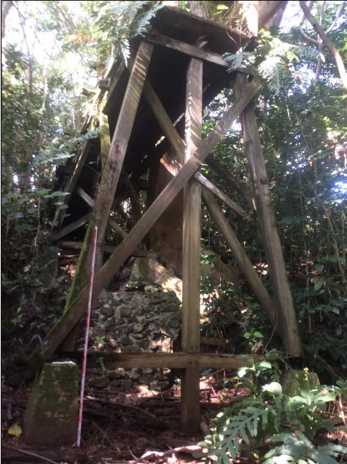
Figure 225. West portion of Feature L, showing support structure including wooden beams, concrete foundations, and mortared basalt retaining walls, view to west
