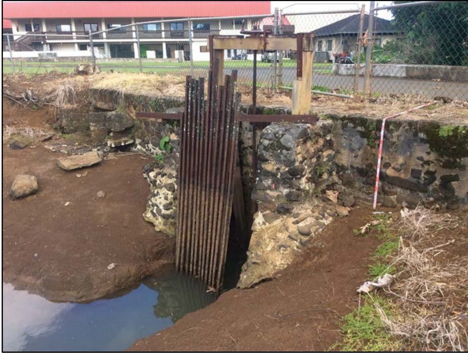
Figure 182. SIHP # -2179 Sub-feature H1, showing retaining wall, sluice gate (right), and flume (left) with lower water level in Feature H, view to northeast
