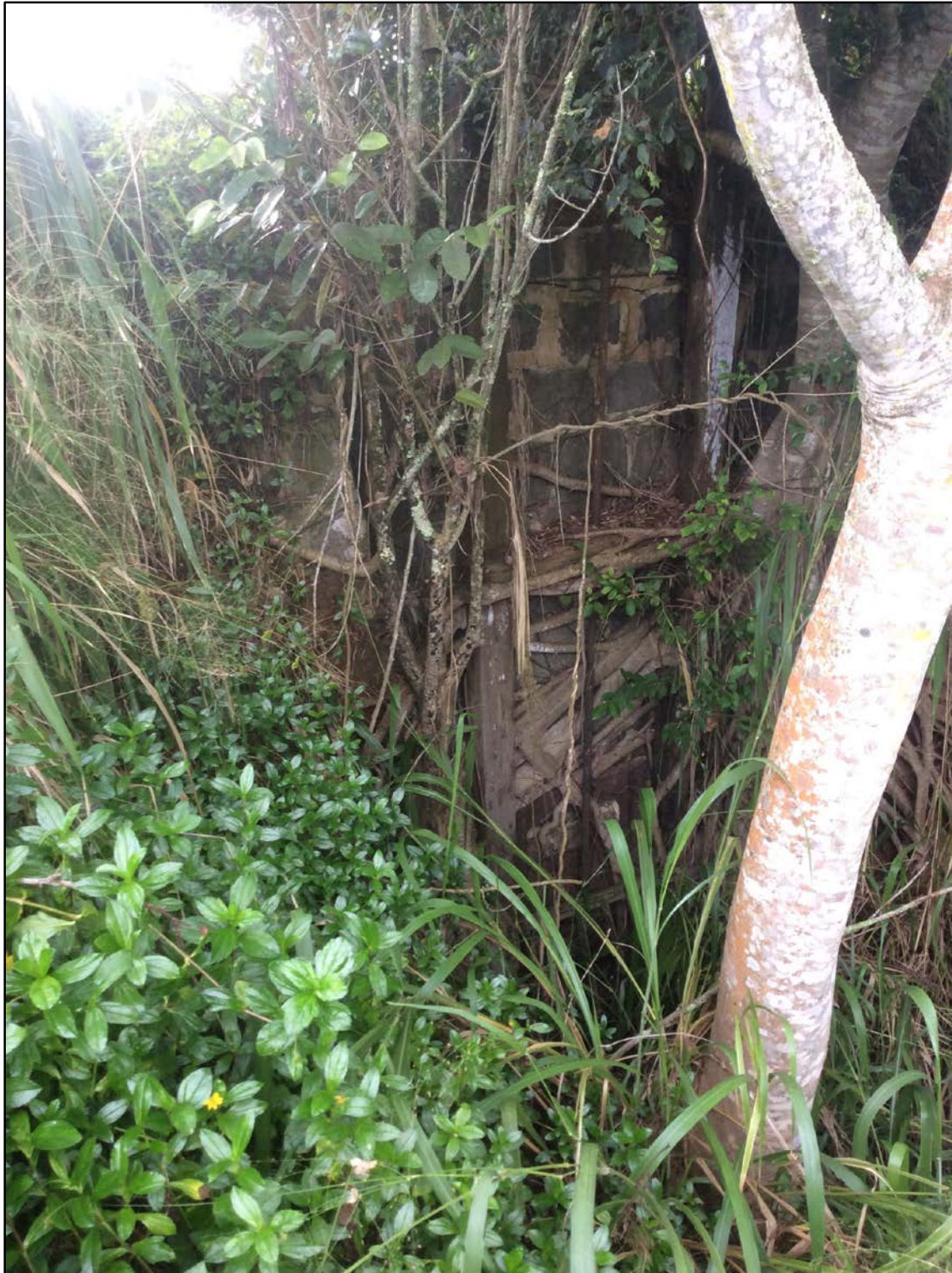
Figure 164. SIHP # -2179 Sub-feature F1 showing mortared basalt retaining wall and wooden beam structure holding sluice gate, view to southeast
