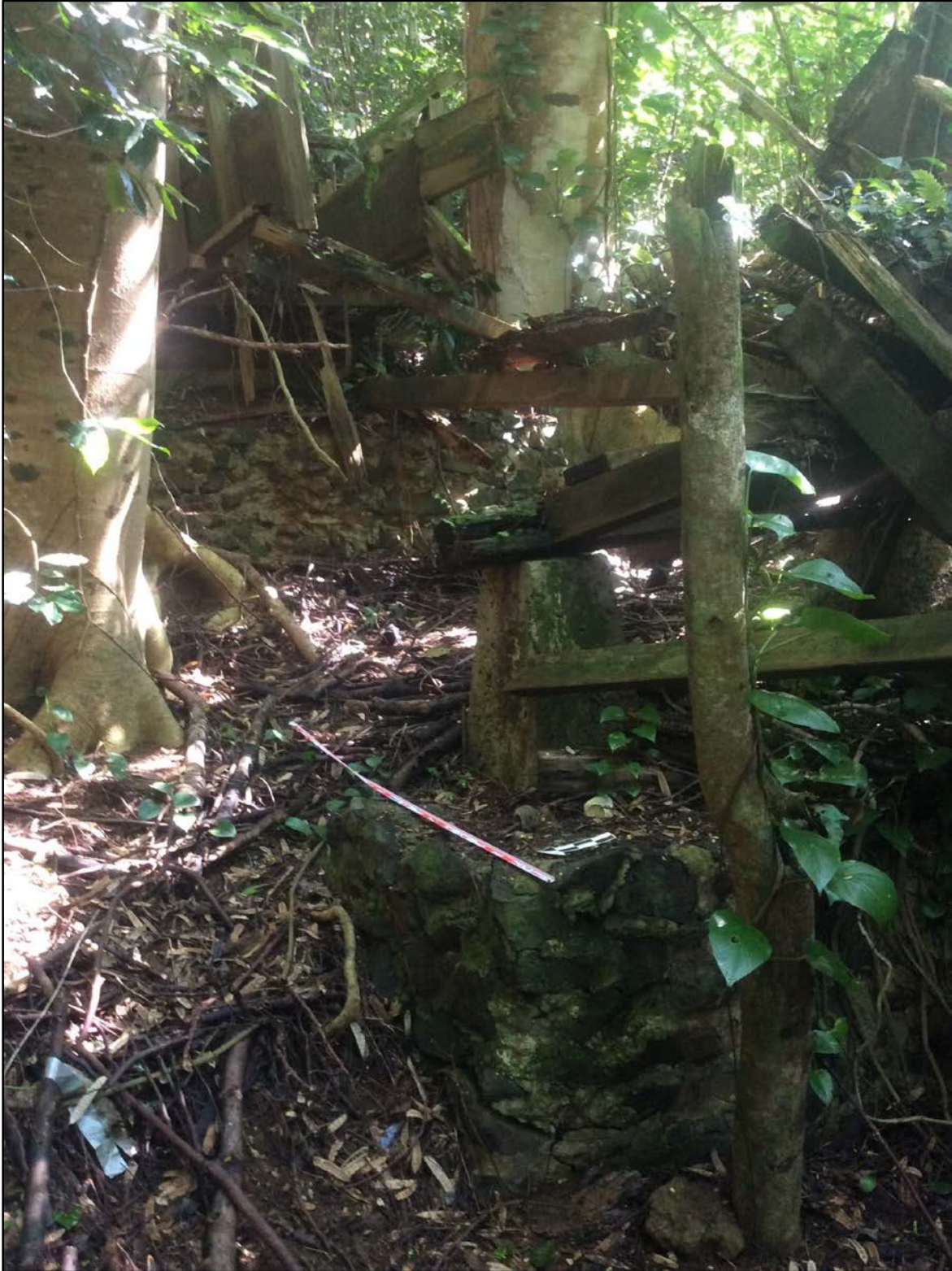
Figure 230. Remnants of support structure of east portion of Feature L including wooden beams, concrete foundations, and mortared basalt retaining walls, view to southeast
