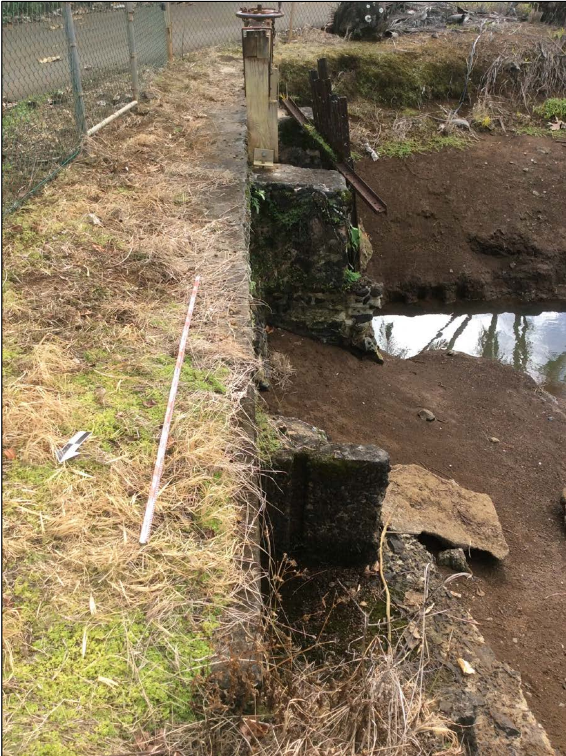
Figure 181. SIHP # -2179 Sub-feature H1, retaining wall, view to south
