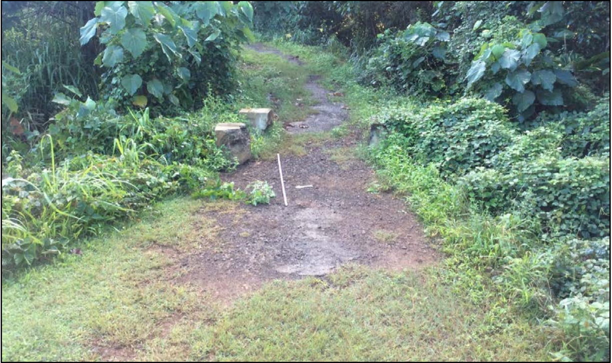
Figure 204. View of roadway above Sub-feature I4, showing patches of asphalt, view to east
