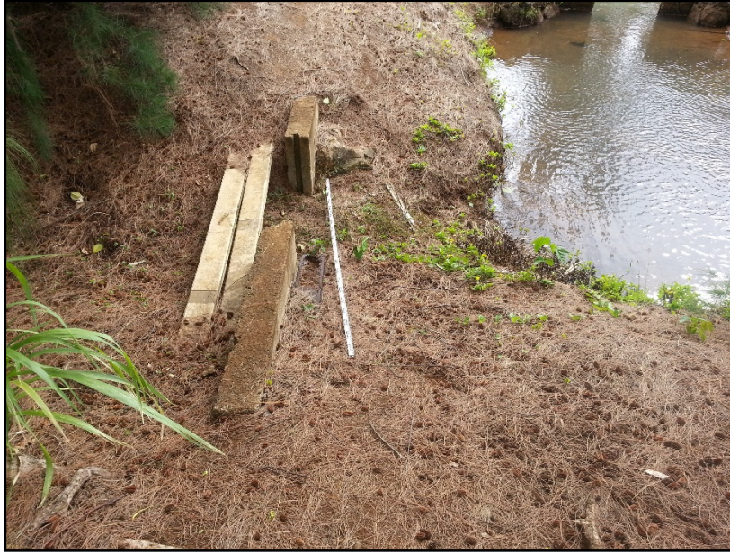
Figure 107. Photo of SIHP # -2179 Feature A2, sluce gate at the easternmost edge of the Feature A overflow area, view to south (Hunkin et al. 2014)
