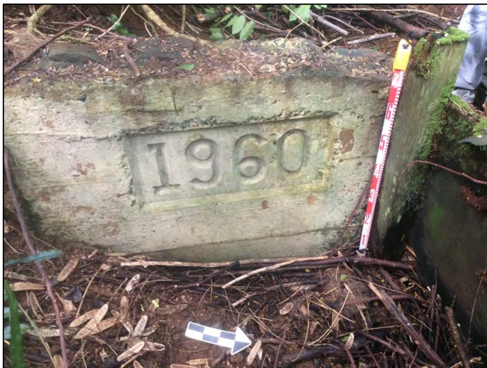
Figure 223. Sluice gate foundation with date “1960,” view to west
