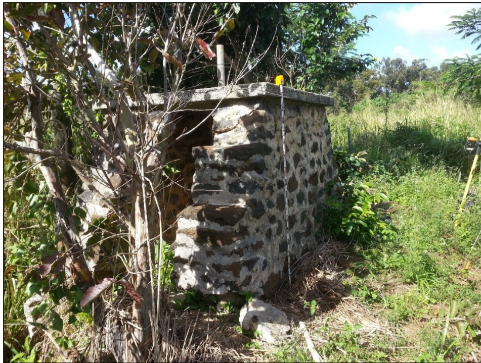
Figure 287. Photo of SIHP # -2220, showing the overall structure, including the trapezoid-shaped walls, the steps on the east wall, the square concrete slab topping the structure, and the metal pipe protruding outward from the top
