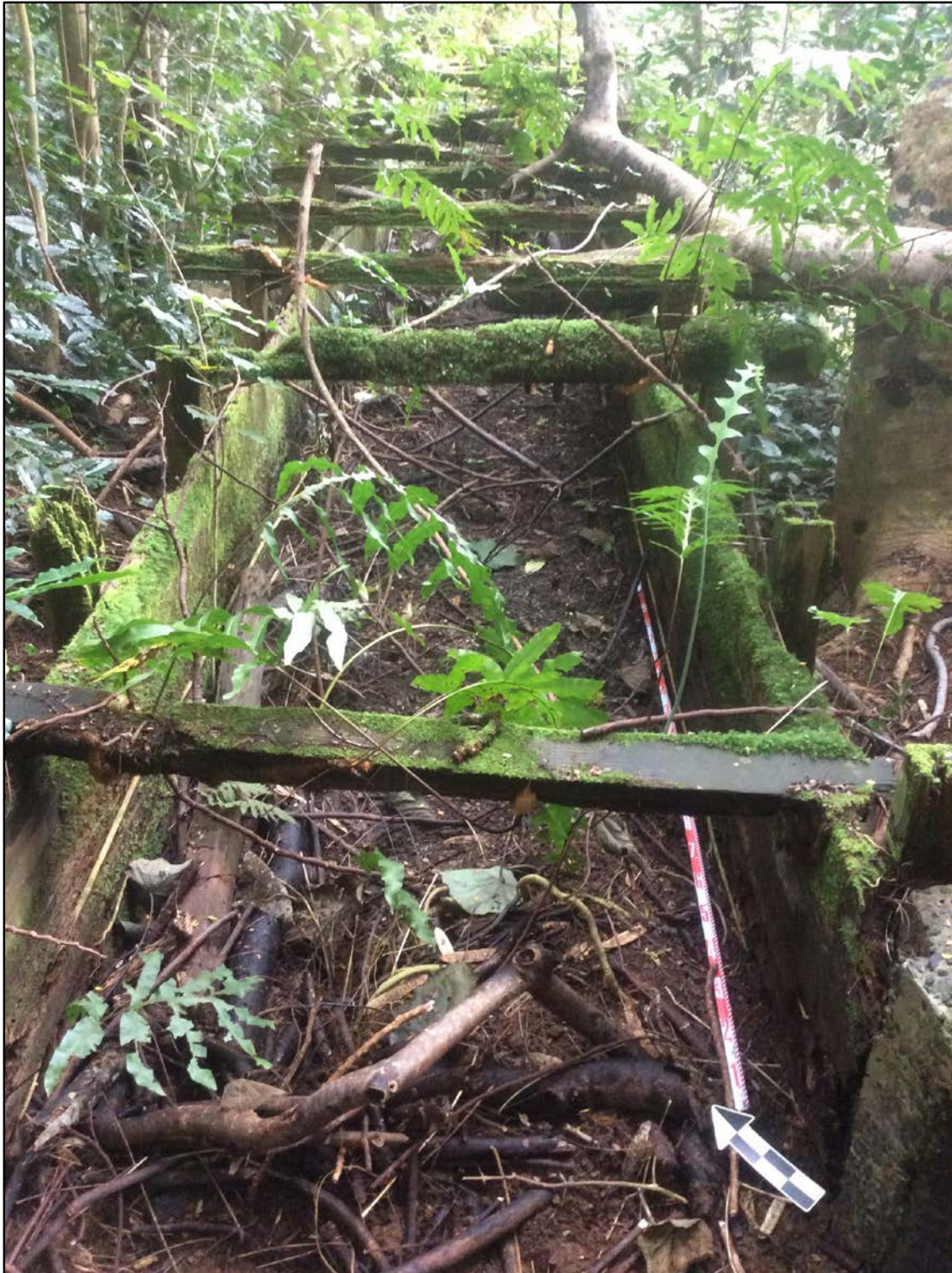
Figure 224. West portion of Feature L, showing general construction design, view to northeast
