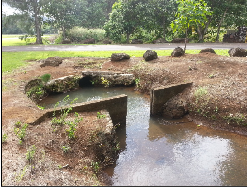
Figure 109. Photo of SIHP # -2179 Feature A3, sluice gate at the southwest side of the Feature A overflow area, water flows through the pipe in background, under the Island School road, into Feature F, irrigation ditch, view to southwest (Hunkin et al. 2014)
