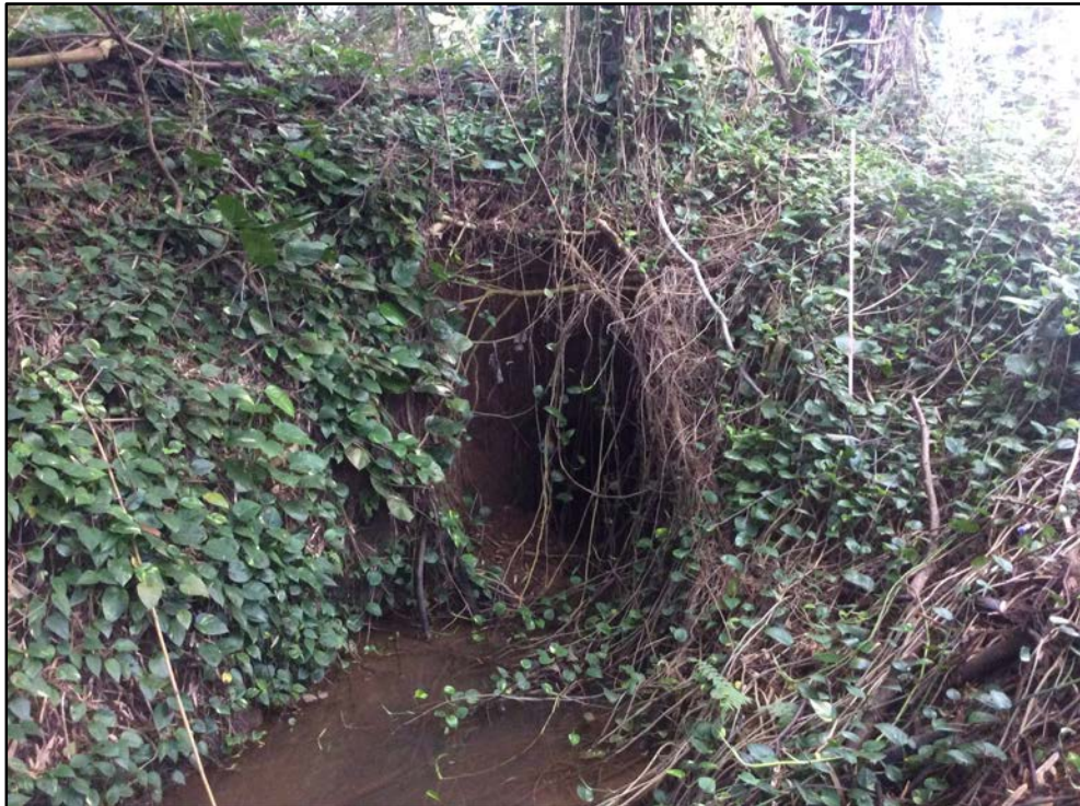
Figure 241. Sub-feature M2, irrigation ditch tunnel outflow, view to southwest
