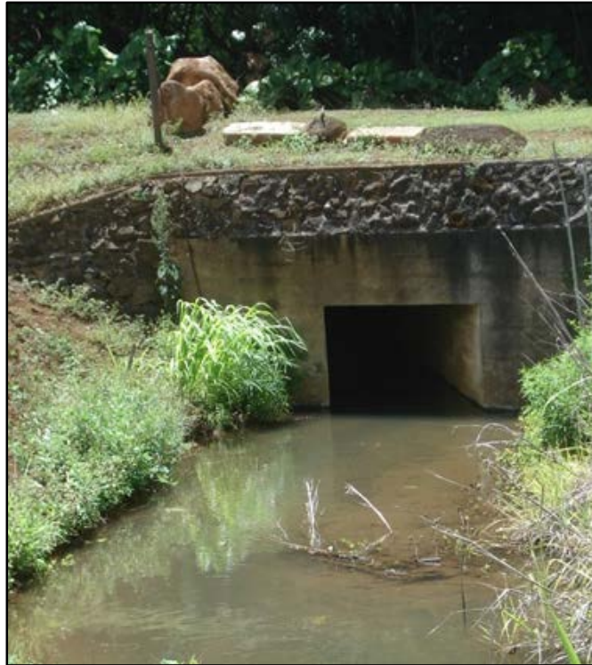
Figure 202. SIHP # -2719 Feature I4, showing concrete culvert and mortared basalt retaining wall, photograph adapted from Groza and Hammatt 2010, view to south
