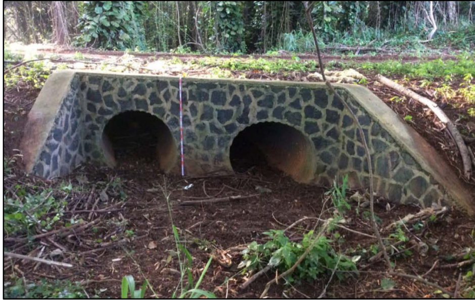
Figure 210. Sub-feature K1, north end of culvert, view to southeast
