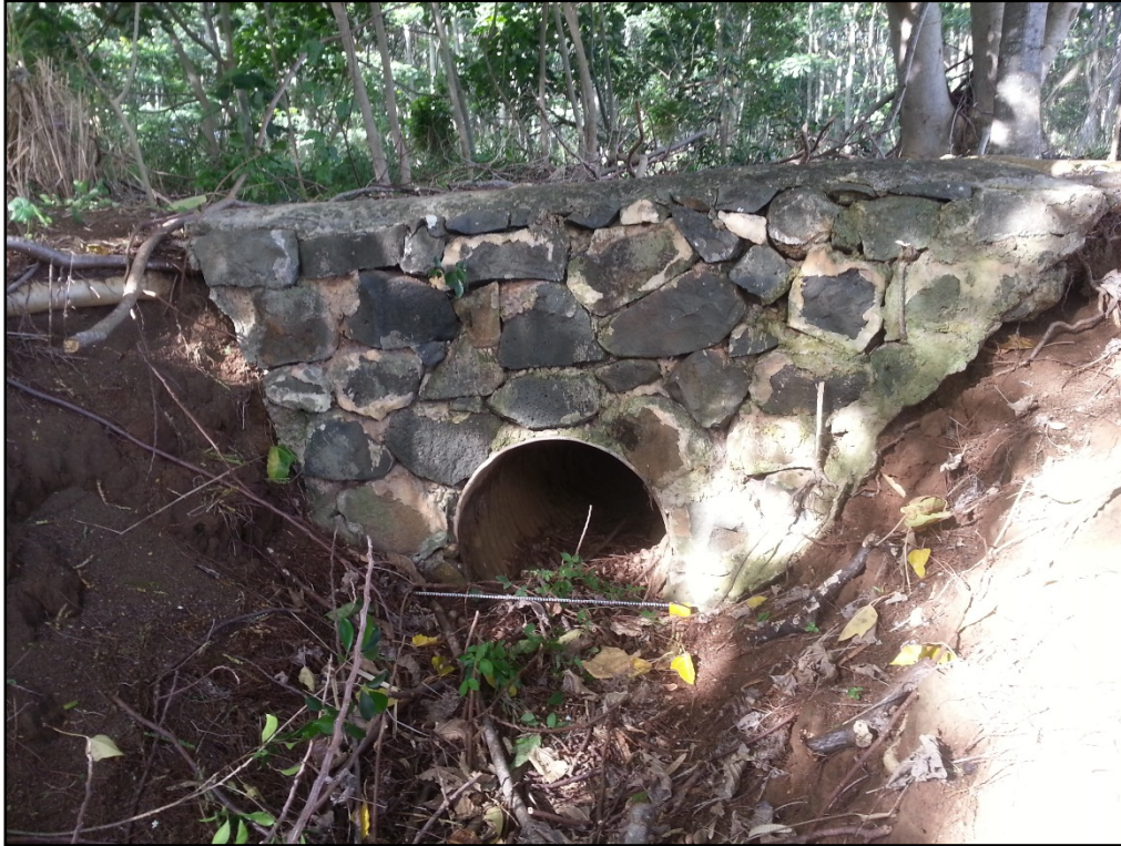
Figure 121. Photo of SIHP # -2179 Feature B1, eastern culvert, view to west (Hunkin et al. 2014)
