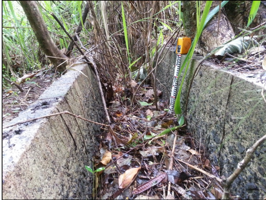
Figure 158. Portion of flume, SIHP # -2179 Feature E1, view to northwest
