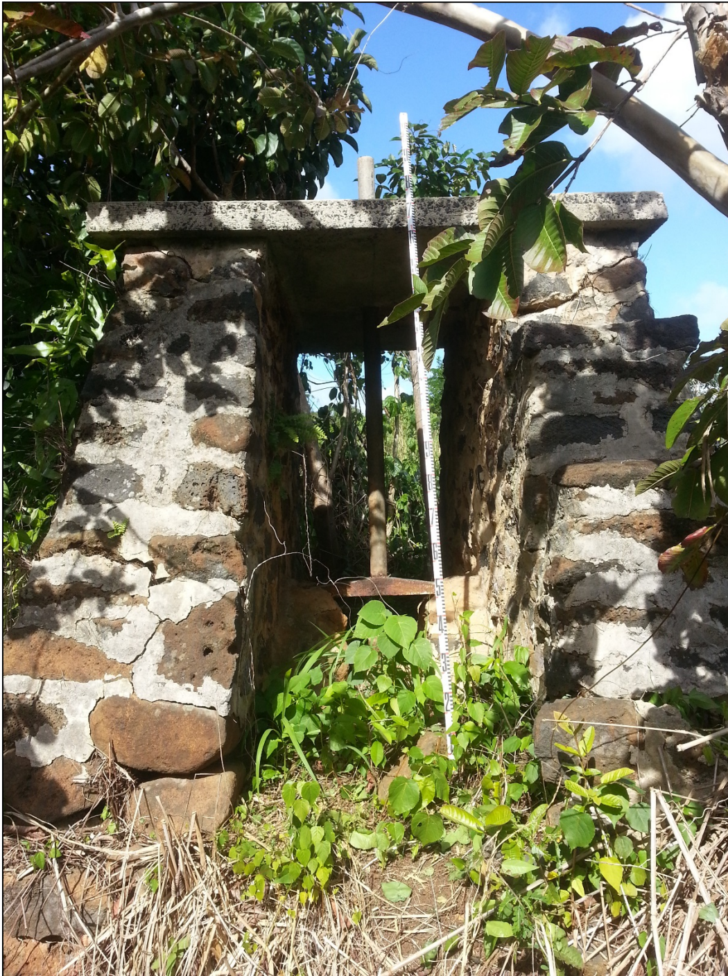
Figure 286. Photo of SIHP # -2220, showing the short protruding inner walls supporting the metal structure with a base and pipe that runs all the way to and through the concrete slab at the top
