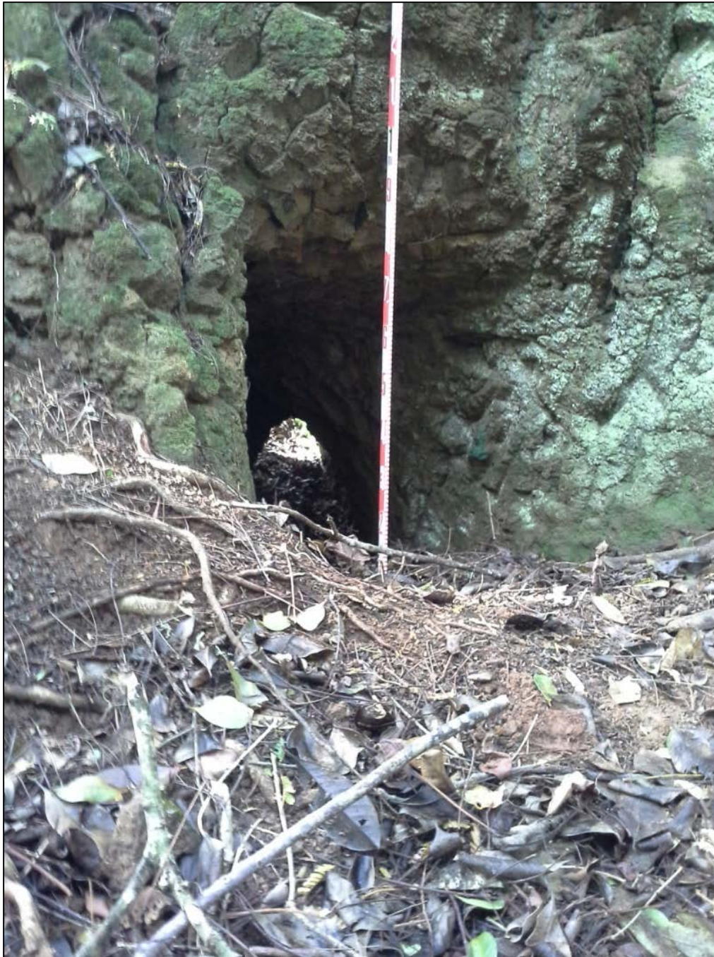
Figure 273. Photo of northwest tunnel opening (Sub-feature P1), southeast opening in the background, view to southeast
