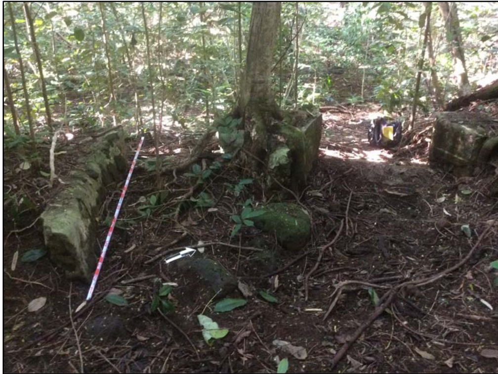
Figure 262. Sub-feature N3, showing two sluice gates, view to northwest
