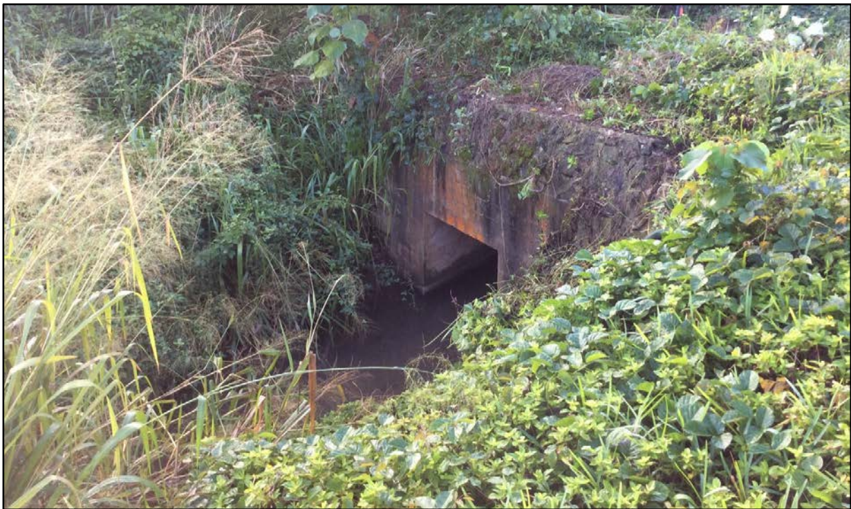
Figure 203. Sub-feature I4, showing current condition of culvert, view to southeast
