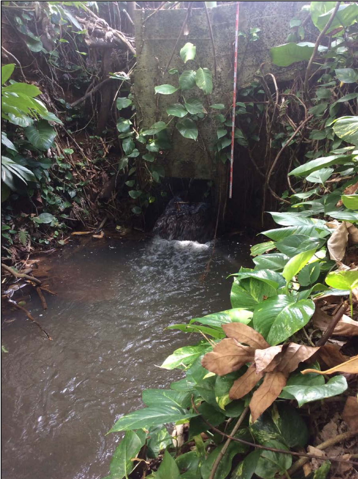
Figure 186. Profile view of sluice gate outtake and flume at the origin of Feature I, irrigation ditch, view to west
