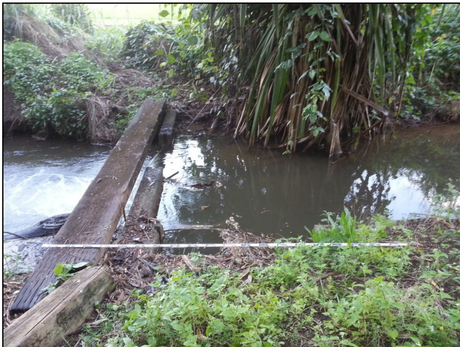
Figure 141. Photo of SIHP # -2179 Feature C4, showing the 4-inch by 12-inch board of treated wood just southwest of (nearly atop) the active gate, view to west (Hunkin et al. 2014)
