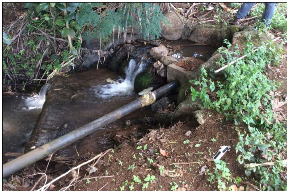
Figure 176. SIHP # -2179 Feature G2, west end of culvert showing modern pipe for diverting and transporting water, view to northwest
