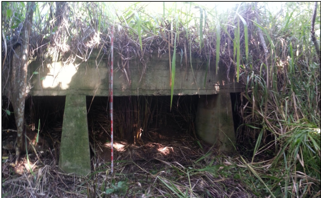
Figure 157. SIHP # -2179 Feature E1, flume, showing concrete footings, view to northwest
