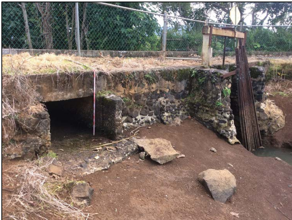
Figure 183. SIHP # -2179 Sub-feature H1, showing retaining wall, sluice gate (right), and flume (left) with lower water level in Feature H, view to southeast
