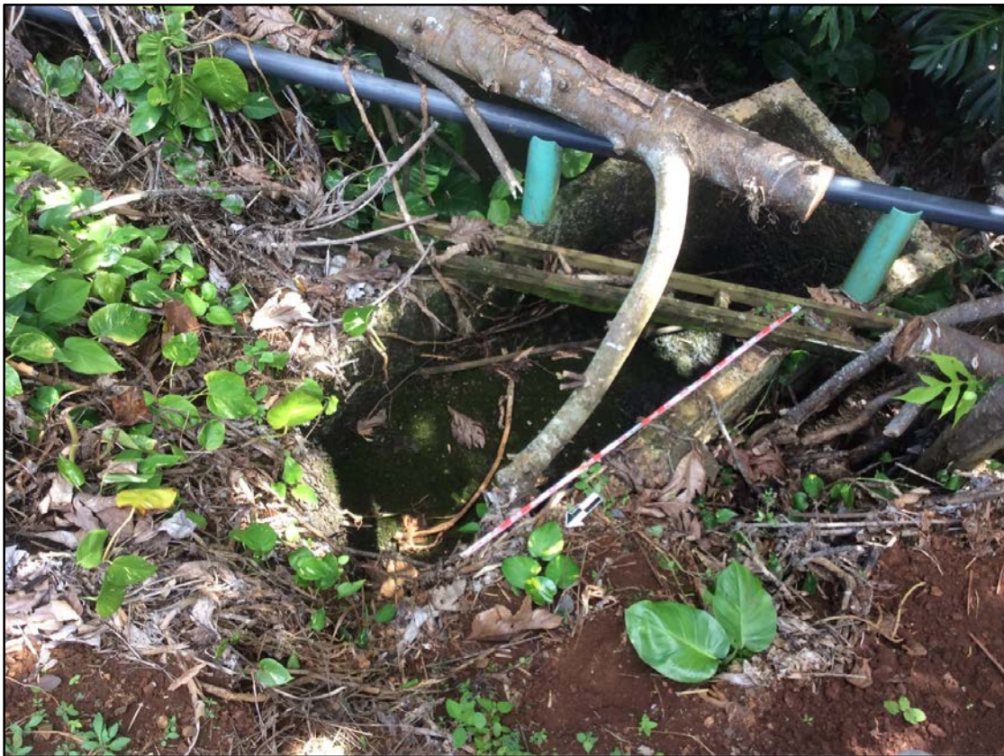
Figure 185. SIHP # -2179 Sub-feature H1, flume on west end of road, view to southeast
