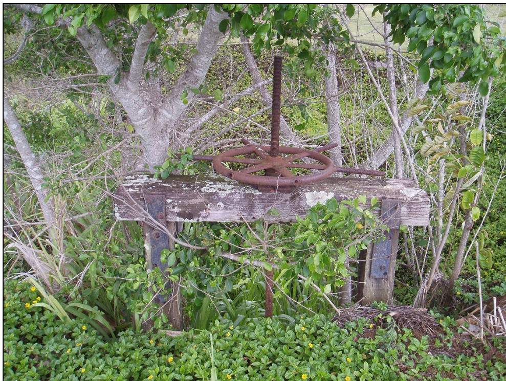
Figure 163. Sluice gate (Sub-feature F1) associated with Feature F, view to north
