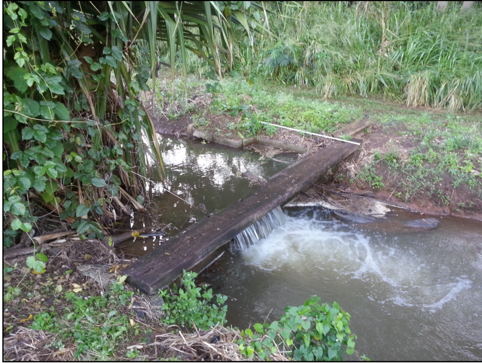
Figure 140. Photo of SIHP # -2179 Feature C4, one active and one abandoned vertical rising sluce gate, view to northwest (Hunkin et al. 2014)
