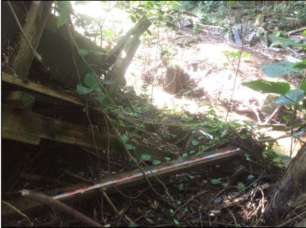
Figure 228. Feature M crossing over central portion of Feature L, collapsed section of east portion in foreground, view to southwest
