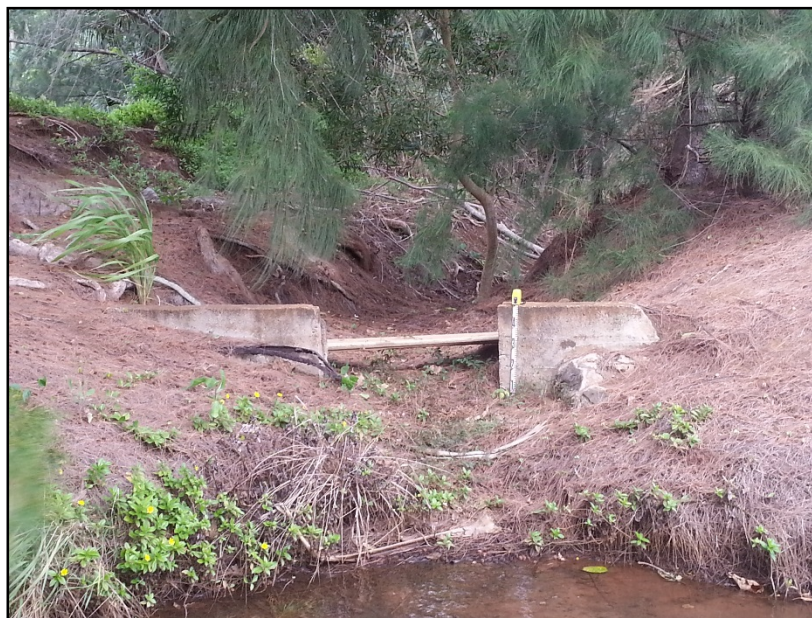
Figure 108. Photo of SIHP # -2179 Feature A2, sluce gate at the easternmost edge of the Feature A overflow area, view to east (Hunkin et al. 2014)
