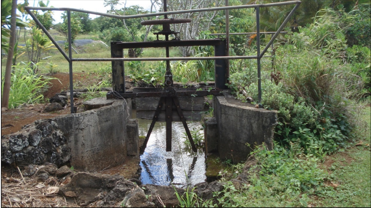
Figure 190. SIHP # -2179 Sub-feature I1, north sluice gate, diverting water to pipe that flows under grass road to Feature J, view to east, photo adapted from Groza and Hammatt 2010 (note wooden bridge over the south sluice gate had not yet been constructed)
