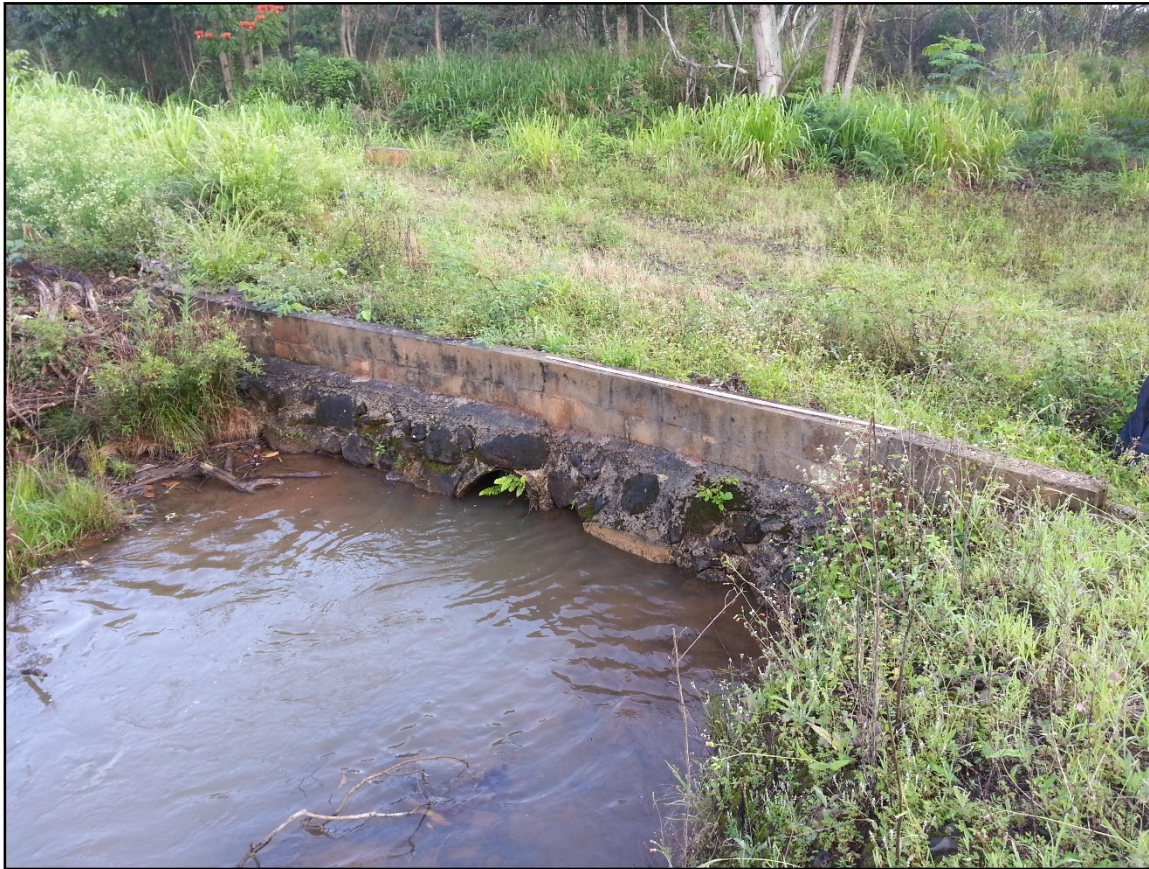
Figure 131. Photo of SIHP # -2179 Feature C1, culvert at northernmost section, view to north (Hunkin et al. 2014)
