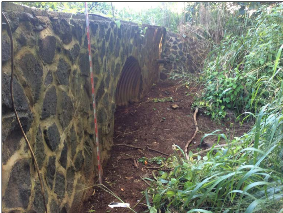
Figure 220. Sub-feature K2, south end showing riprap at east end and metal pipe, view to east
