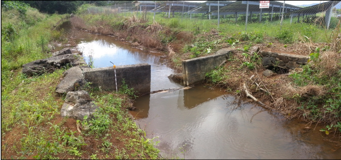
Figure 137. Photo of SIHP # -2179 Feature C3, an abandoned culvert located approximately 0.80 m north of Feature C2, view to southwest (Hunkin et al. 2014)
