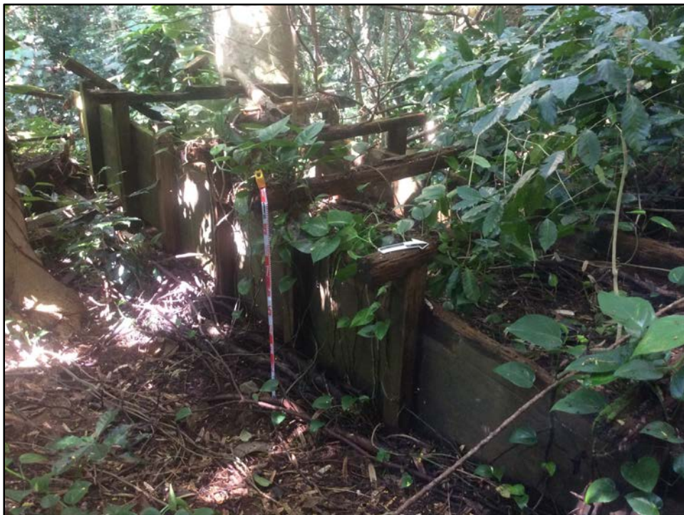
Figure 229. Intact section of east portion, showing general construction, view to west
