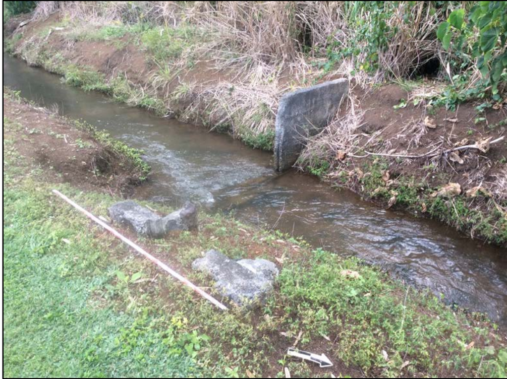
Figure 173. SIHP # -2179 Sub-feature G1, sluice gate remnant, view to west
