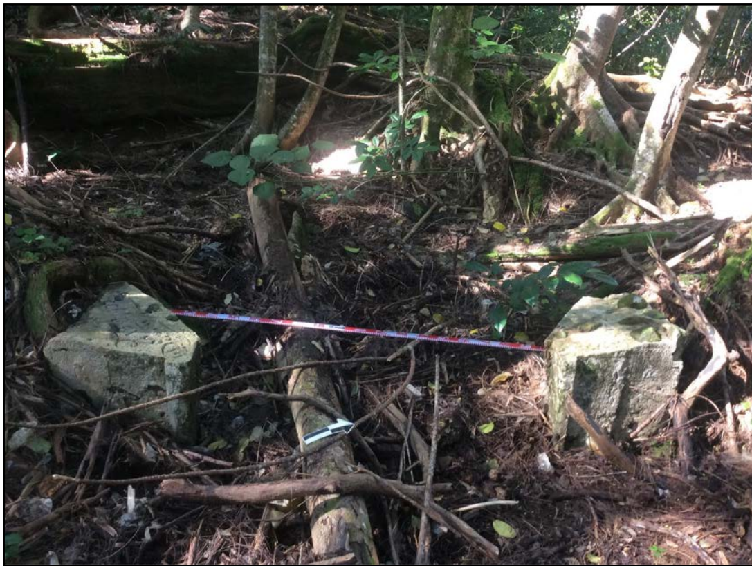
Figure 259. Sub-feature N2, abandoned sluice gate, view to northwest
