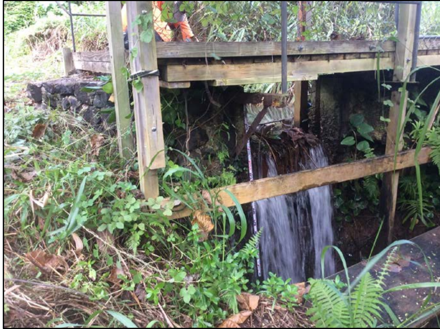
Figure 192. SIHP # -2179 Sub-feature I1, south sluice gate, maintaining water flow through Feature I, view to north
