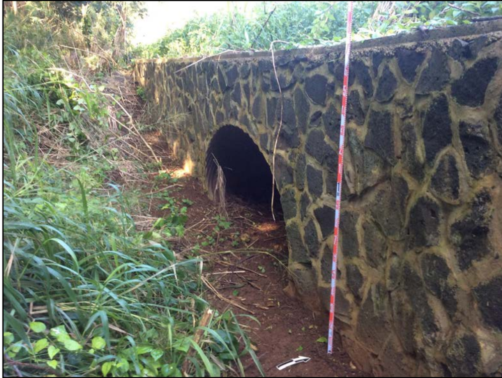
Figure 219. Sub-feature K2, south end showing riprap on west end, view to northwest
