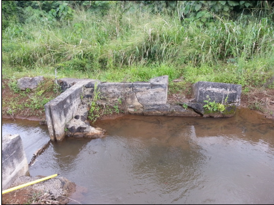
Figure 134. Photo of SIHP # -2179 Feature C2, consisting of one active and one abandoned vertical rising sluice gate, somewhat perpendicular to each other, view to east (Hunkin et al. 2014)
