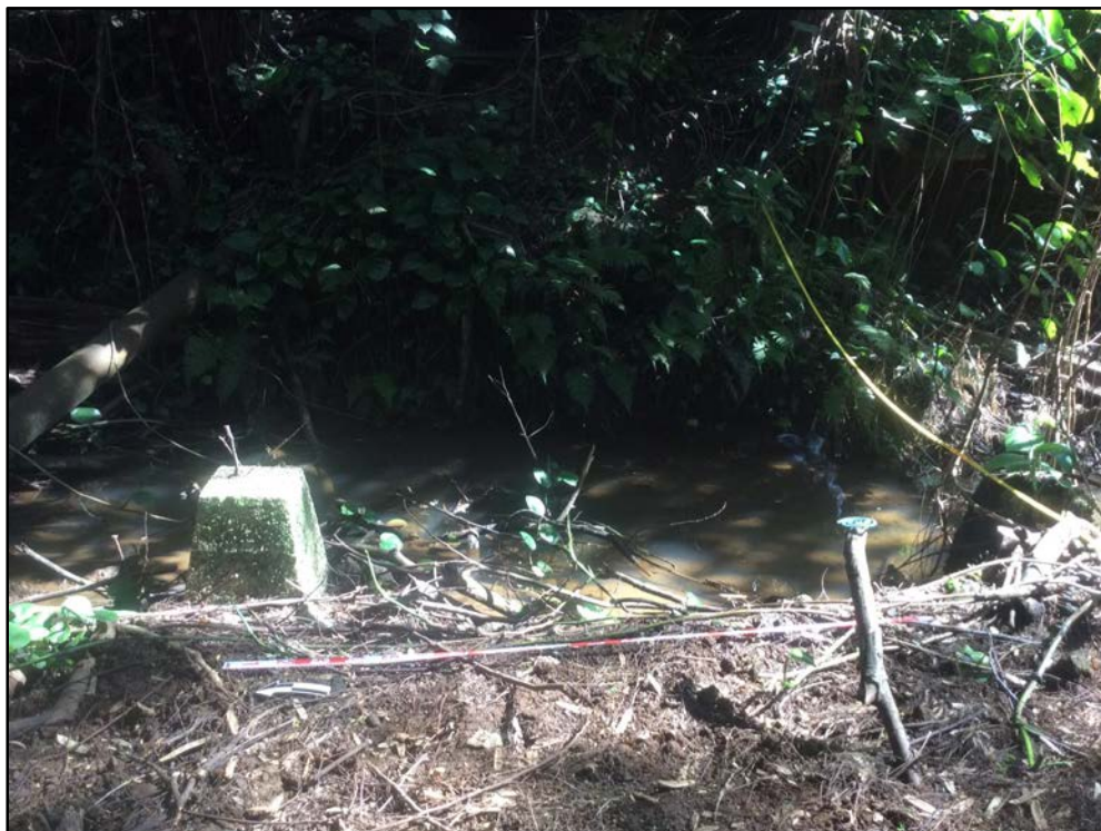
Figure 227. Feature M crossing path of Feature L, note concrete foundations on left and right, view to east
