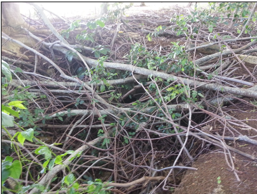
Figure 122. Photo of SIHP # -2179 Feature B1, western culvert, view to east (Hunkin et al. 2014)
