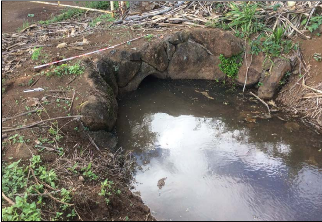
Figure 177. SIHP # -2179 Feature G2, east end of culvert, view to west
