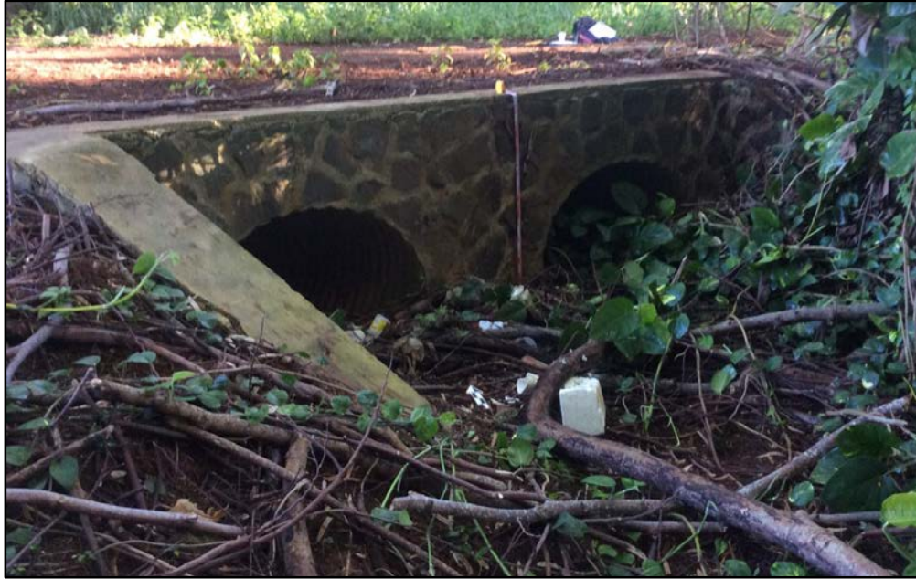
Figure 212. Sub-feature K1, south end, view to northeast
