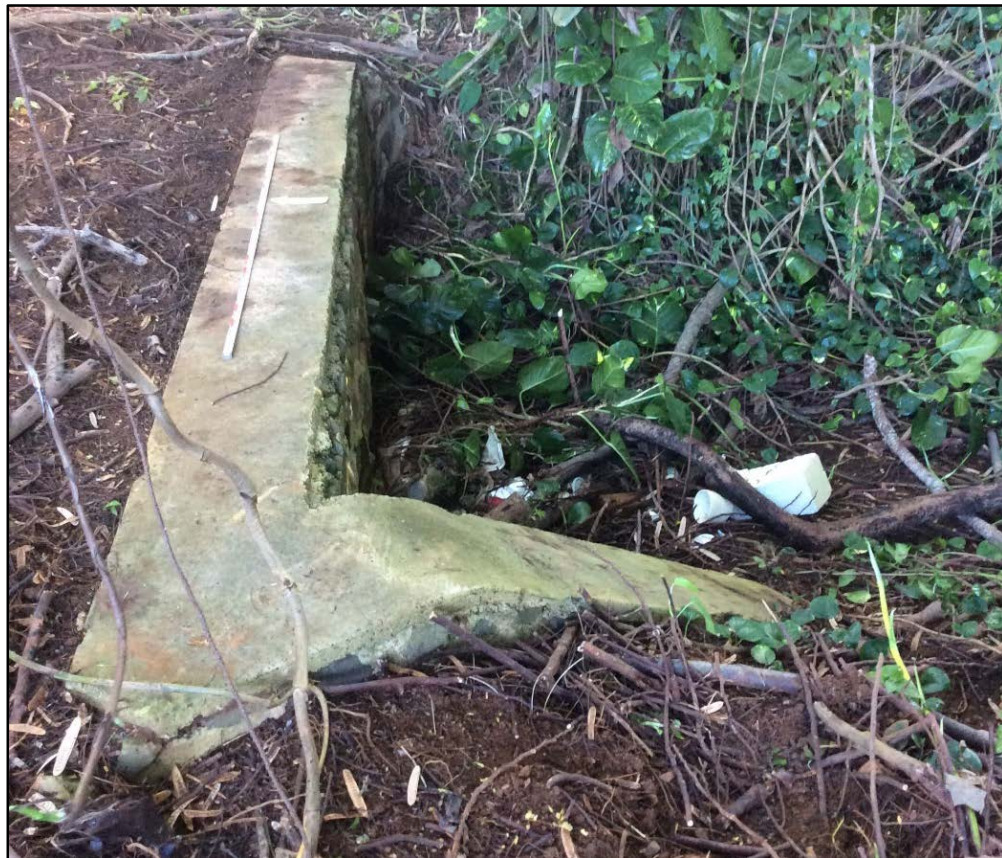
Figure 213. Plan view of Sub-feature K1, south end, view to east
