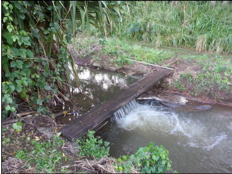
Figure 114. Photo of SIHP # -2179 Feature C4, one active and one abandoned vertical rising sluice gate, view to northwest
