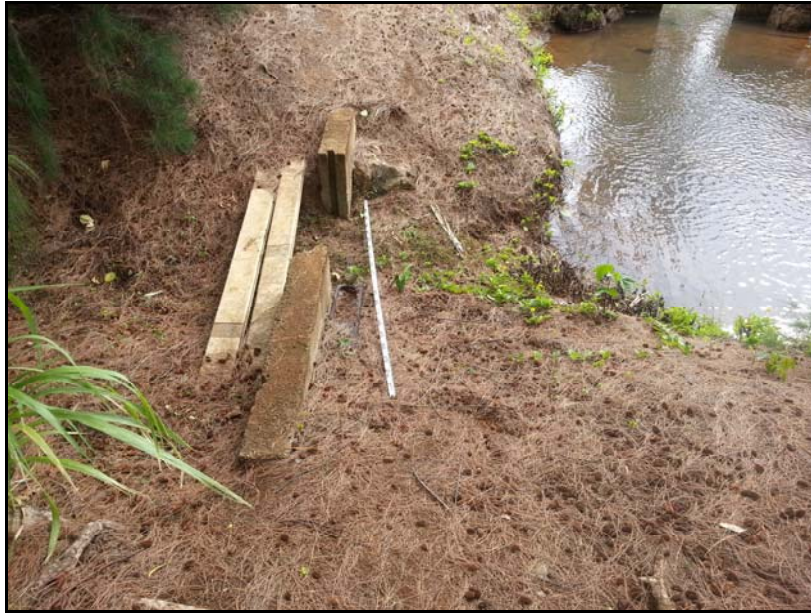
Figure 81. Photo of SIHP # -2179 Feature A2, sluice gate at the easternmost edge of the Feature A overflow area, view to south
