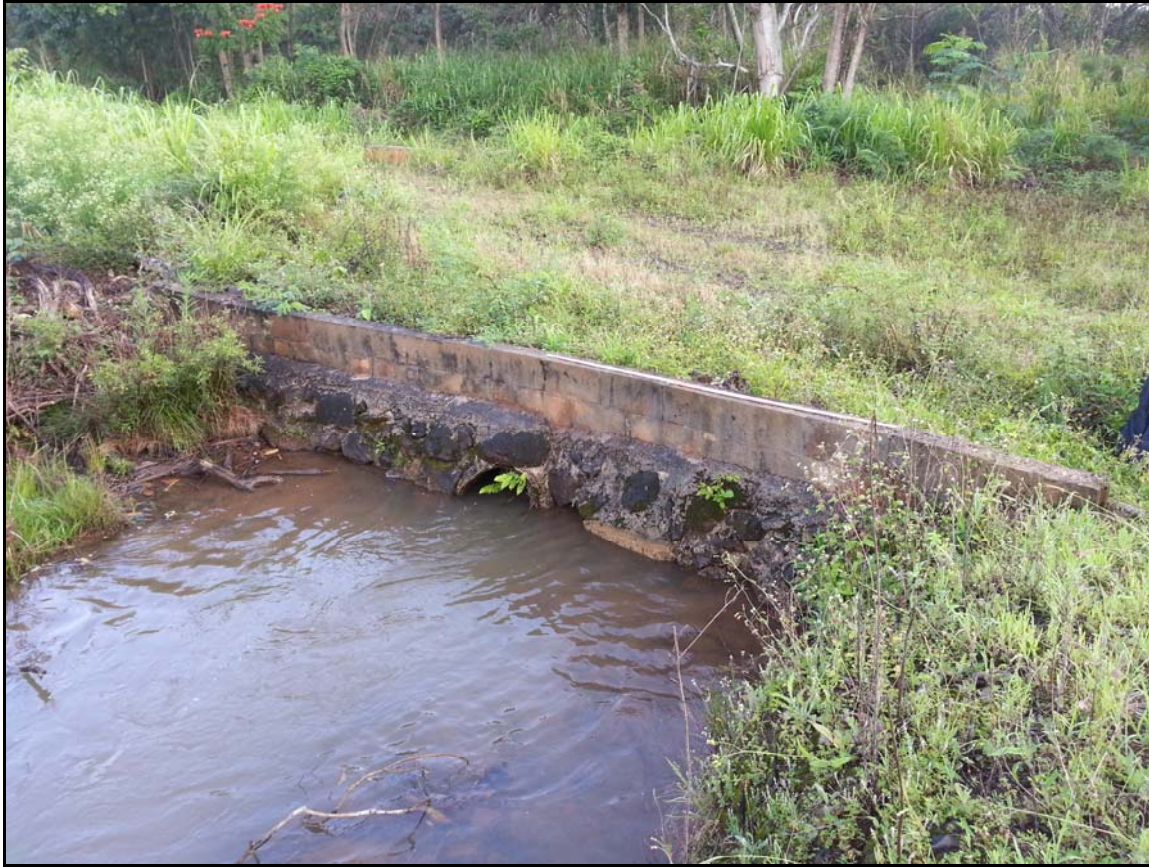
Figure 105. Photo of SIHP # -2179 Feature C1, culvert at northernmost section, view to north
