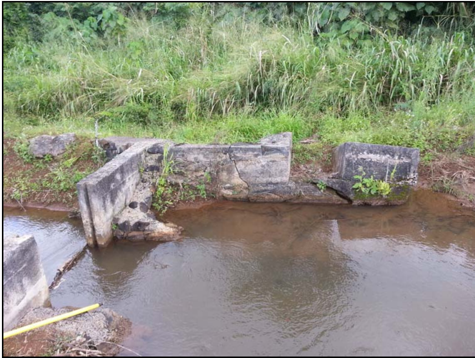
Figure 108. Photo of SIHP # -2179 Feature C2, consisting of one active and one abandoned vertical rising sluice gate, somewhat perpendicular to each other, view to east
