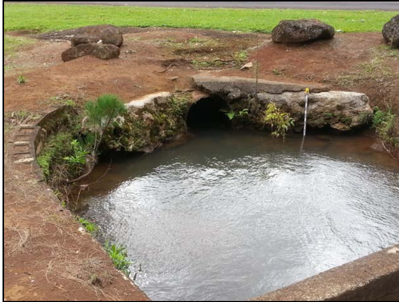
Figure 85. Photo of SIHP # -2179 Feature A4, modern culvert at the south end of the Feature A overflow area, view to southwest
