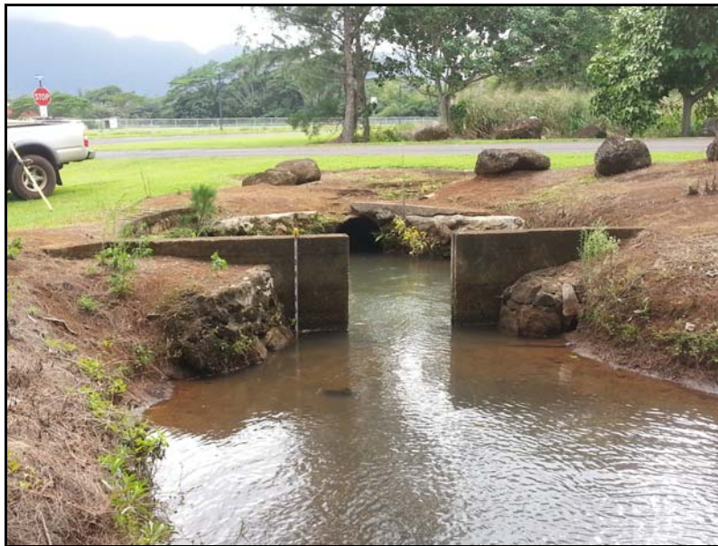
Figure 84. Photo of SIHP # -2179 Feature A3, sluice gate at the southwest side of the Feature A overflow area, view to south
