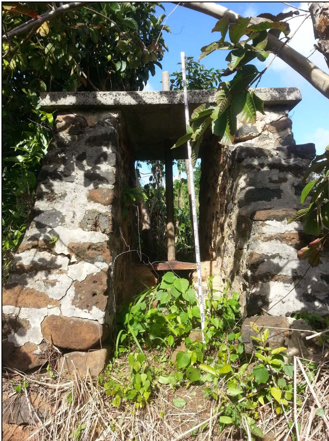
Figure 127. Photo of SIHP # -2220, showing the short protruding inner walls supporting the metal structure with a base and pipe that runs all the way to and through the concrete slab at the top
