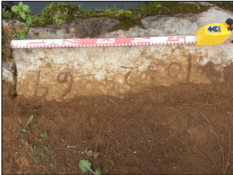
Figure 86. Photo of SIHP # -2179 Feature A4, modern culvert, showing the inscription reading “10-29-69,” view down
