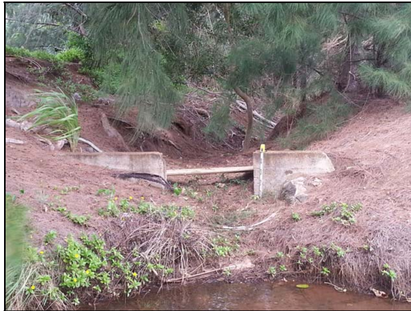
Figure 82. Photo of SIHP # -2179 Feature A2, sluice gate at the easternmost edge of the Feature A overflow area, view to east
