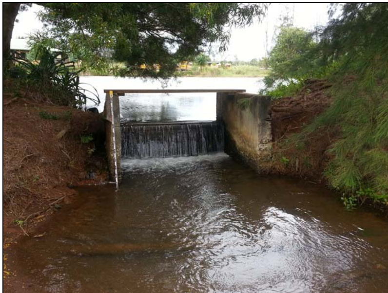
Figure 80. Photo of SIHP # -2179 Feature A1, sluice gate at the northern end of the overflow area, view to north
