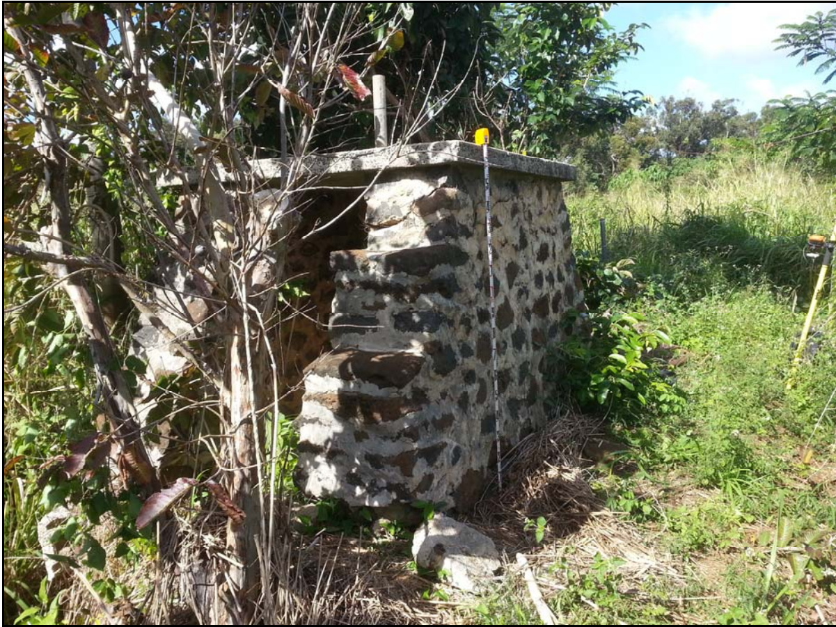
Figure 126. Photo of SIHP # -2220, showing the overall structure, including the trapezoid-shaped walls, the steps on the east wall, the square concrete slab topping the structure, and the metal pipe protruding outward from the top
