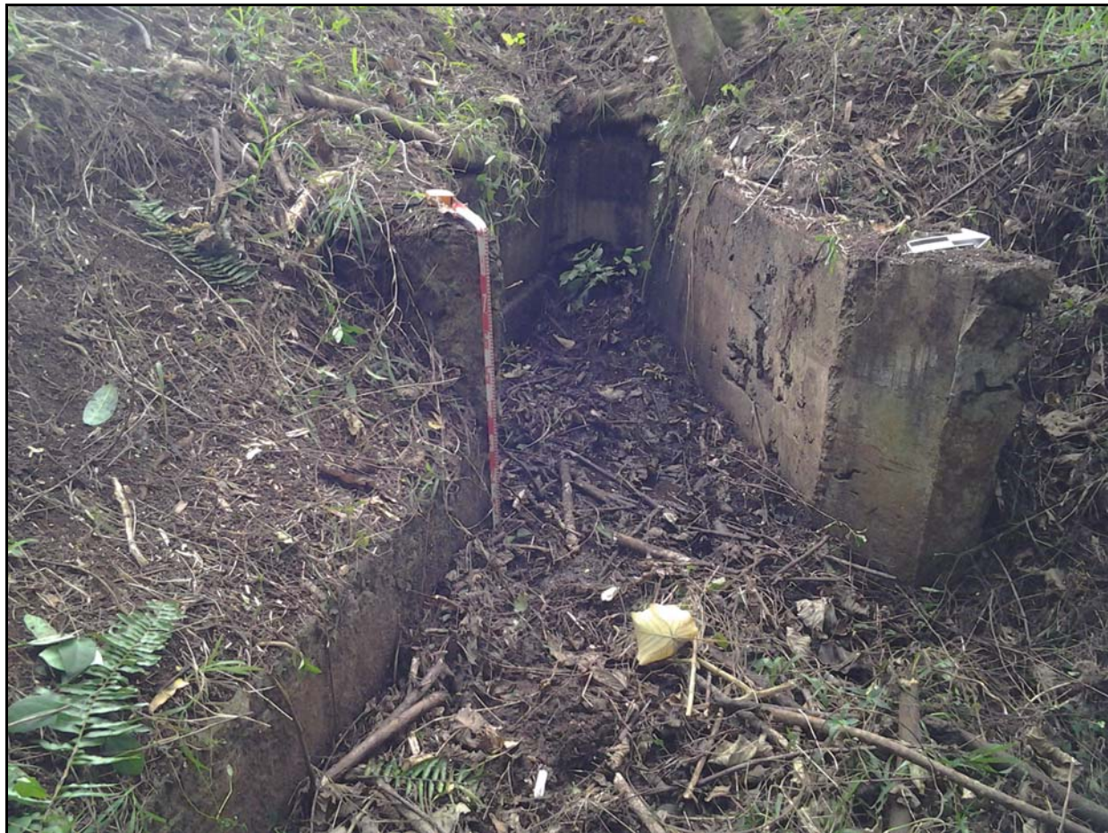
Figure 123. Photo of SIHP # -2179 Feature D1, outlet at the westernmost end of Feature D, which indicates that water from Feature A was diverted and fed into Feature D to be transported to feed cane fields to the east (slightly down slope from Feature C and Feature A), the original Lihue Plantation Company's cane field 39A, view to west
