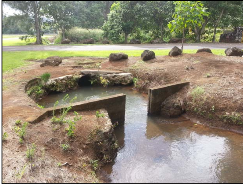
Figure 83. Photo of SIHP # -2179 Feature A3, sluice gate at the southwest side of the Feature A overflow area, view to southwest
