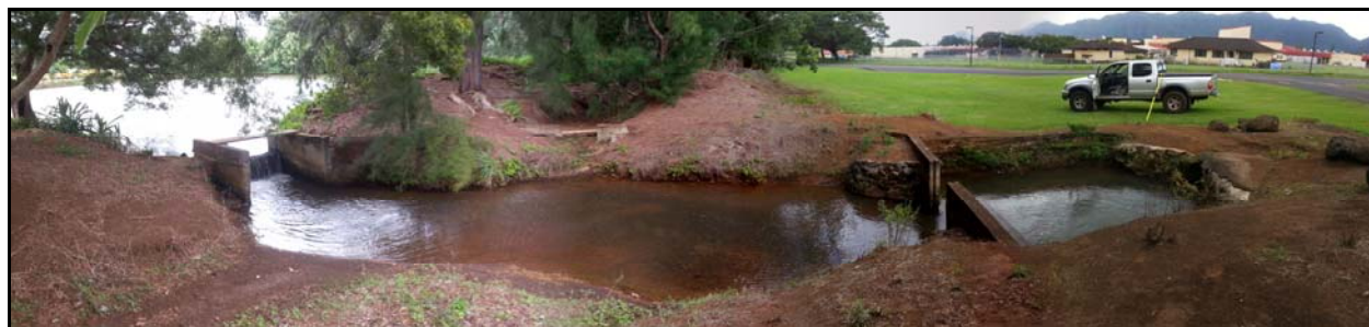
Figure 77. Photo of the overflow area of SIHP # -2179 Feature A, including the four sub-features (Features A1–A4)
