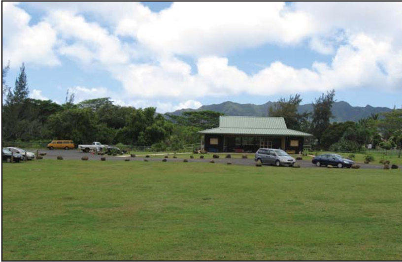
Photo 5: Culture and Arts building within the south-central portion of the Island School campus.
