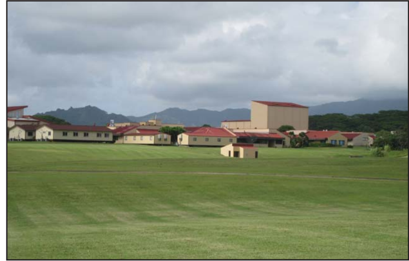
Photo 10: Kaua'i Community College campus from Kaumuali'i Highway looking northwest.
