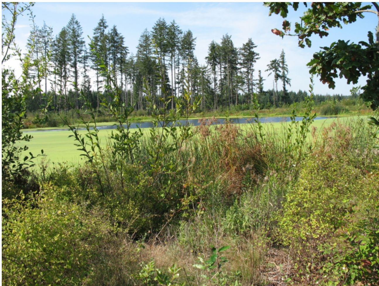
Figure 8-2. A Constructed Wetland for Polishing Treatment and Wildlife Habitat
