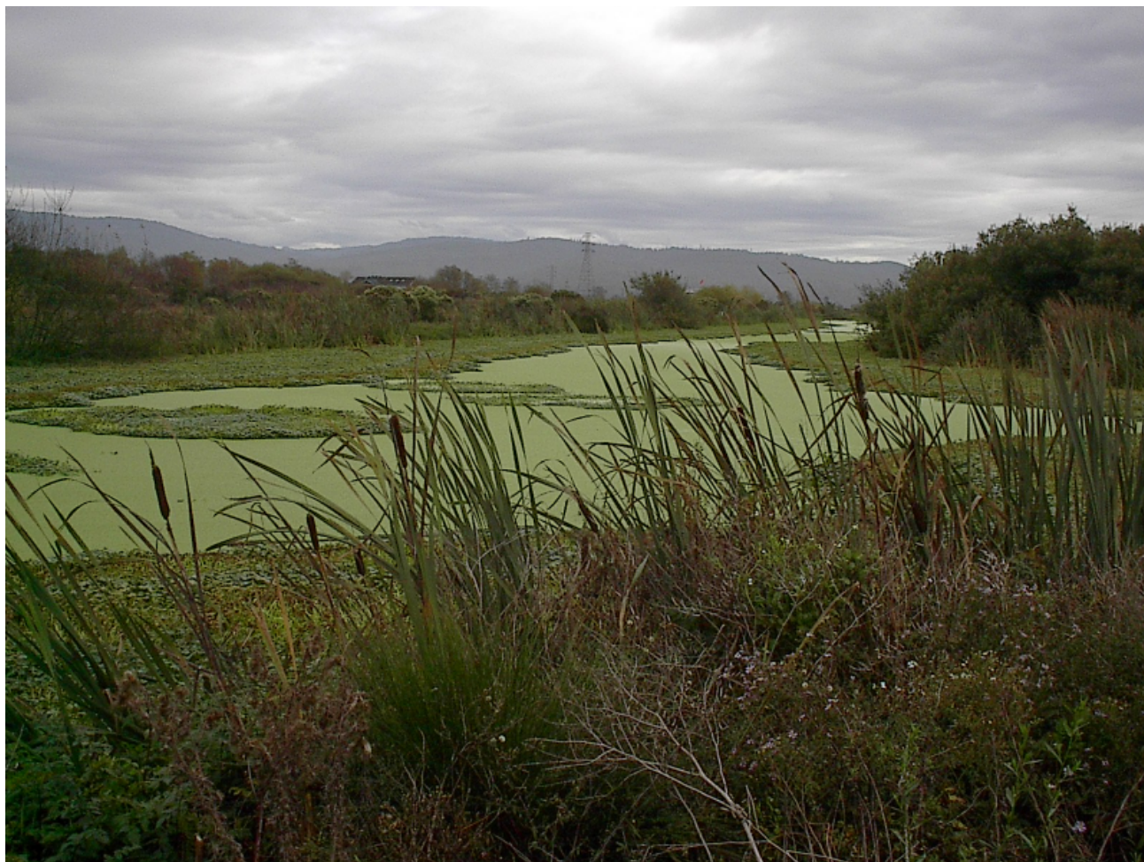
Figure 1-1. A Constructed Wetland for Wastewater Treatment
