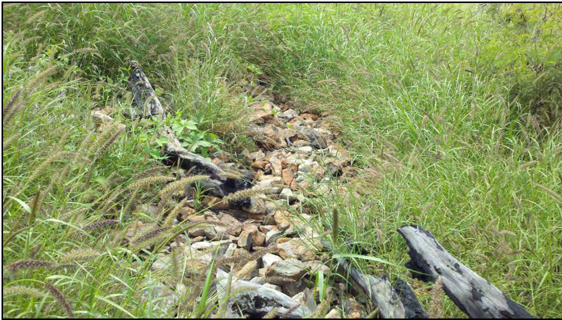
Figure 43. CSH-1, close up showing construction material. View to west.
