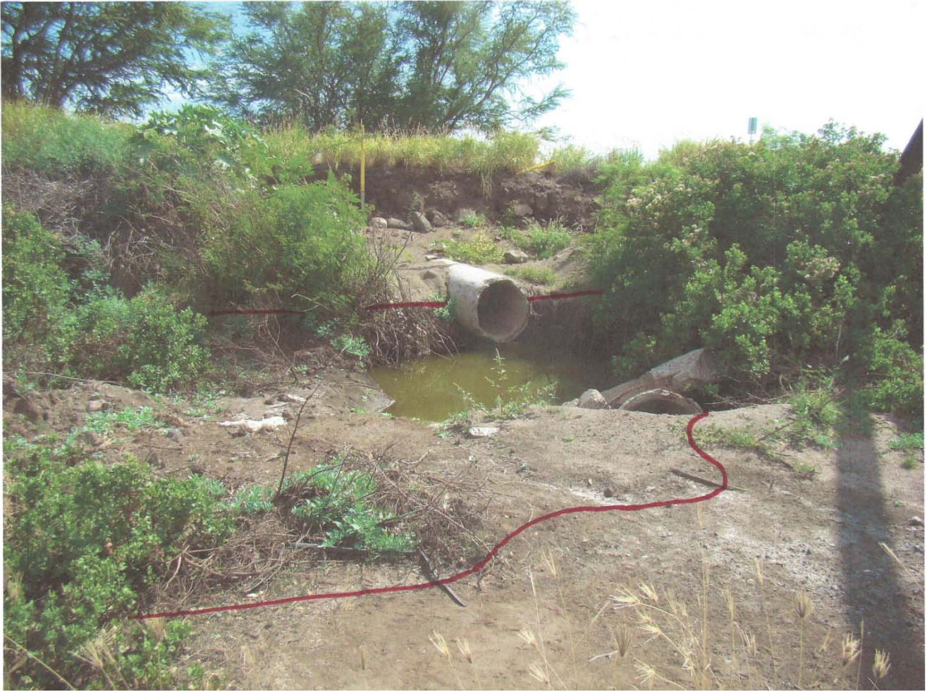
6b A 24 inch culvert running from a highway drainage ditch under Honoapiilani Hwy to the shoreline near the southern most tip of the Project.
