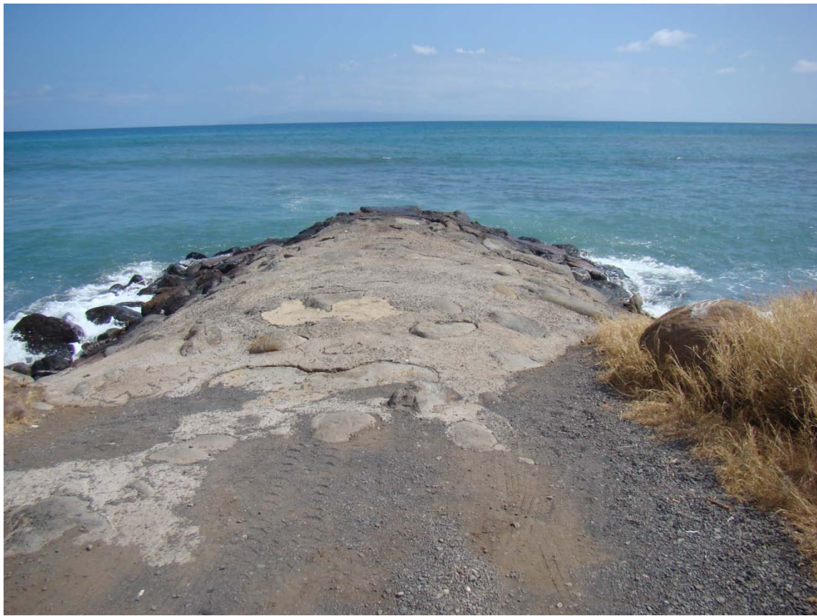
5e Kapaiki Fishpond armored drainage pipe running out into the ocean.
