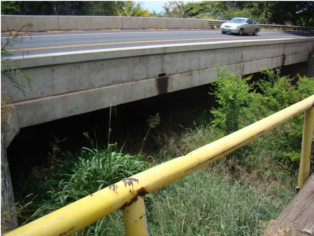
3c Olowalu stream bridge along Honoapiilani Highway showing the span of the box culvert
