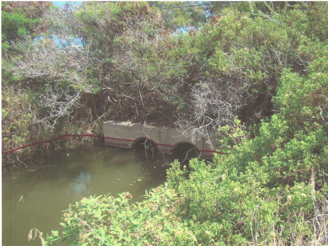
#4 b View makai along Kapaiki Village Drainage Channel where water enters two 24 inch culverts that run under Honoapiilani Highway towards the ocean. OHWM shown.
