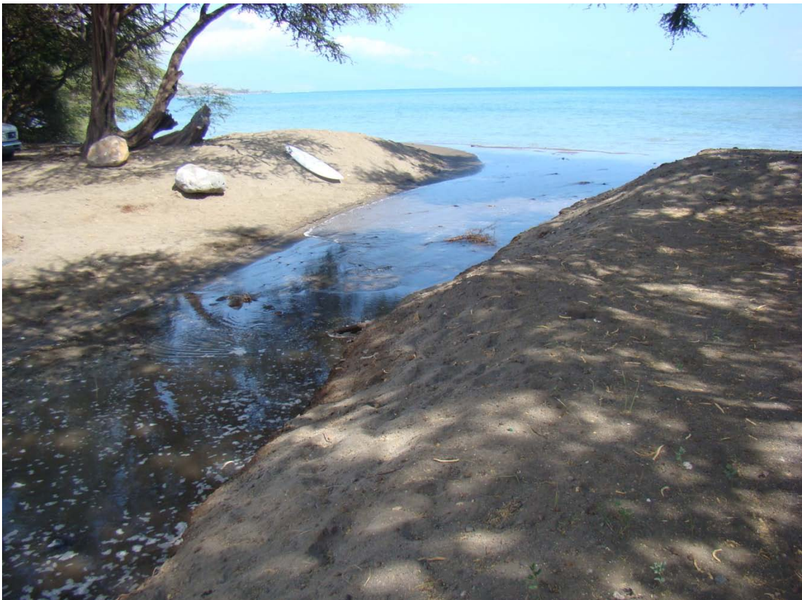
#4 d Kapaiki Village Drainage Channel connection to the ocean showing a Small wave washing into the channel at high tide.
