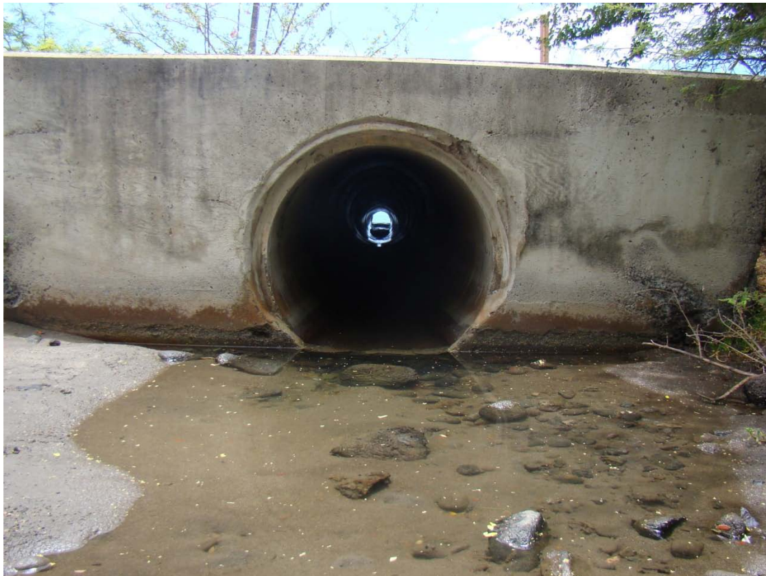
5d Kapaiki Fishpond drainage pipe running under Honoapiilani Highway to the ocean.
