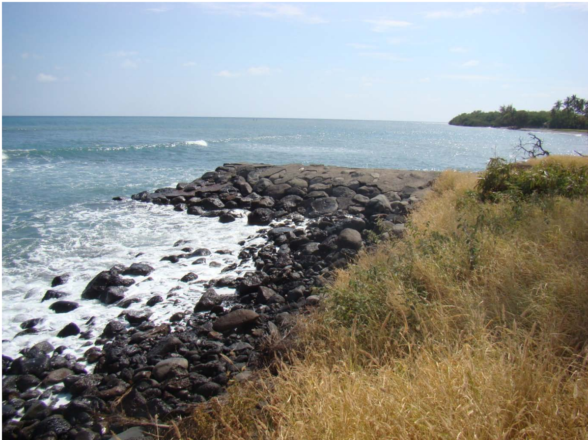
5f Kapaiki Fishpond armored drainage pipe running out into the ocean.
