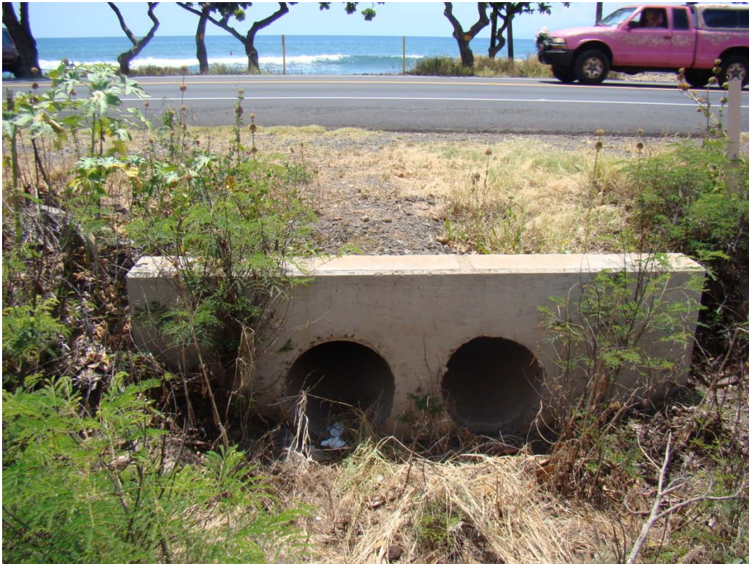
#1 – b Two 24 inch culverts drain a small coastal plain under Honoapiilani Highway
