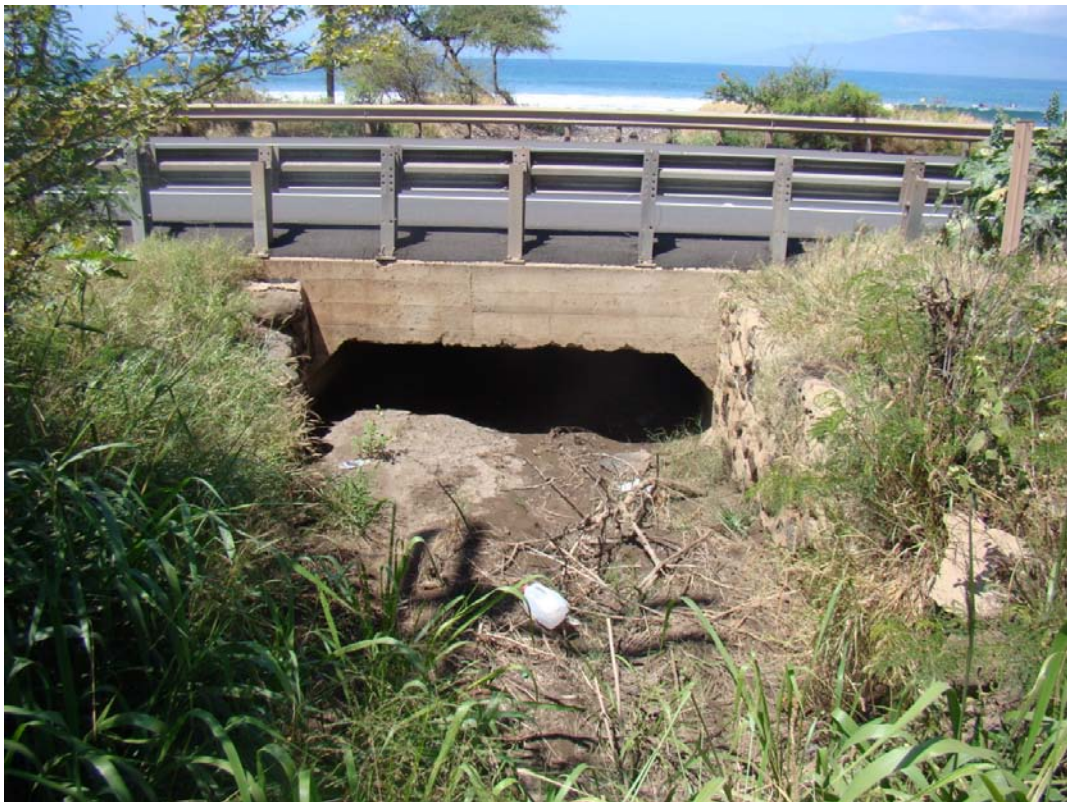
#2d Combined flow from all seven gulches runs through this box culvert and under Honoapiilani Highway
