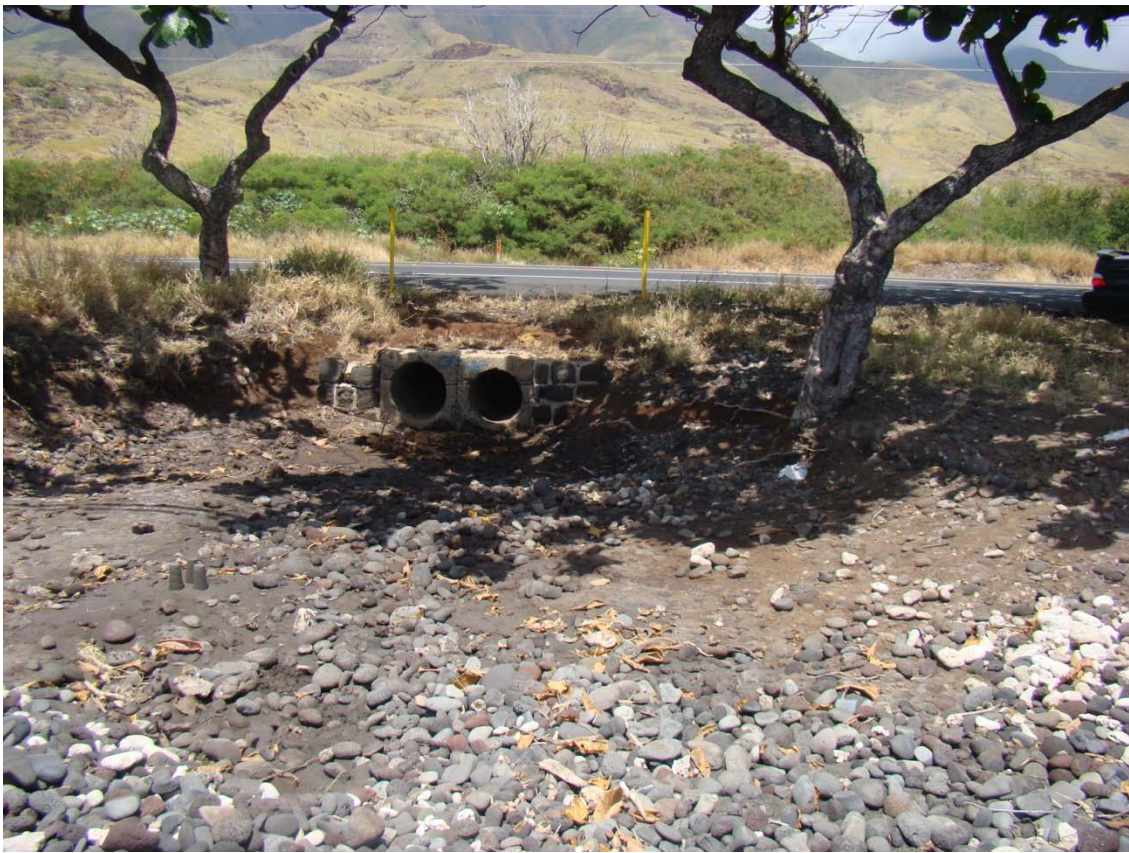
#1 – c Culverts deliver water to rocky shoreline
