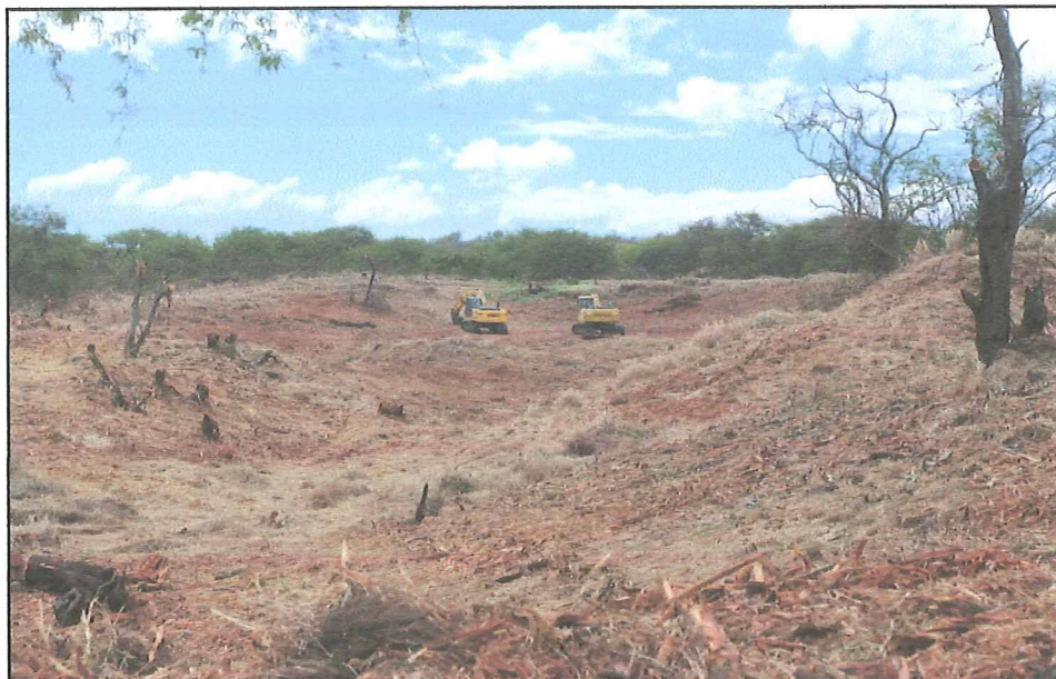
A view towards the south after clearing operations. Photo taken 10/13/14.
