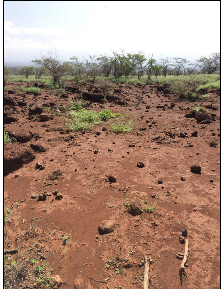
Photo 18: General condition of the waterline easement area.
