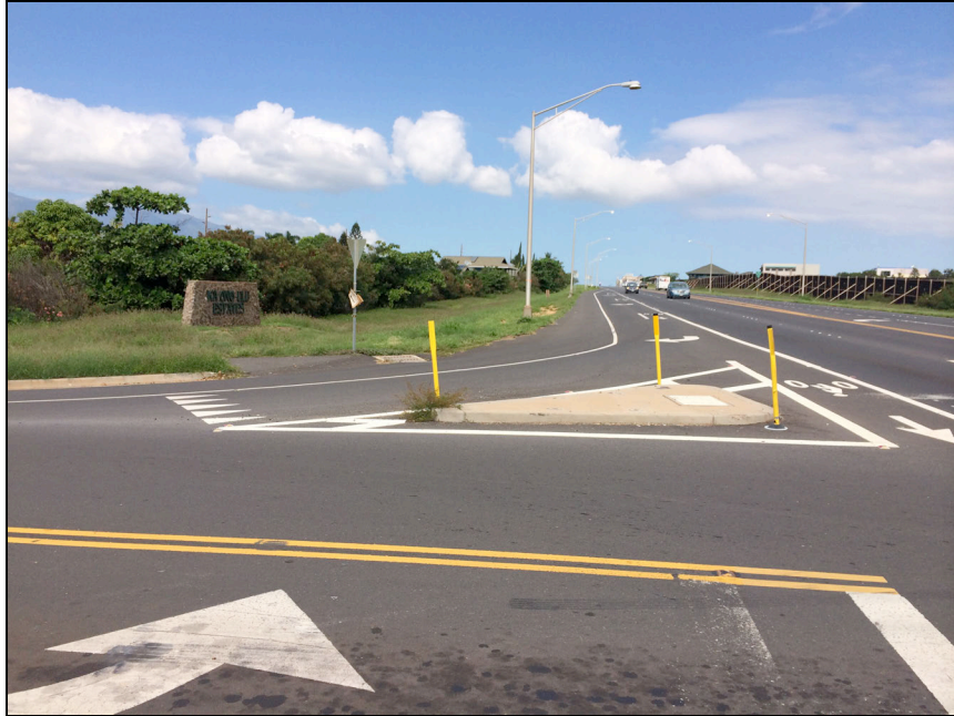
Photo 15: Photo of the off-site improvement area, view towards the North. Piilani Promenade Project in view on the right of the highway.
