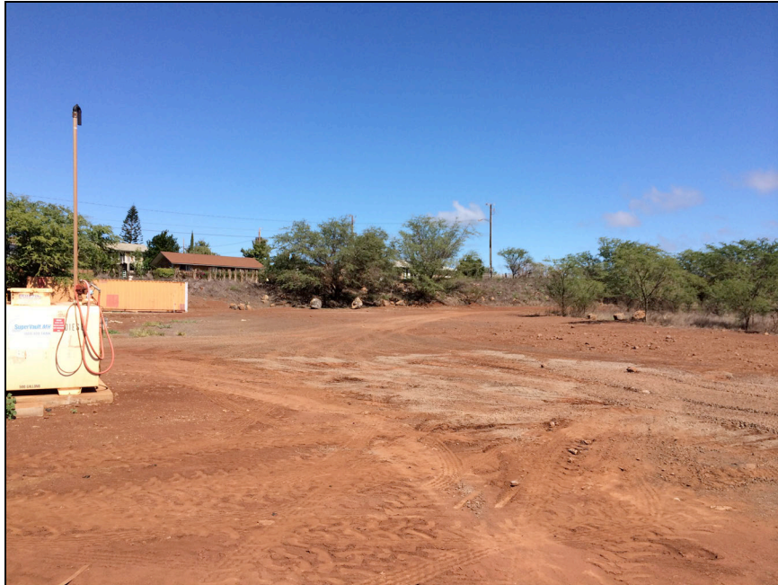
Photo 12: Overview of the Ohukai Access Road – TMK: 2-2-002: 016.
