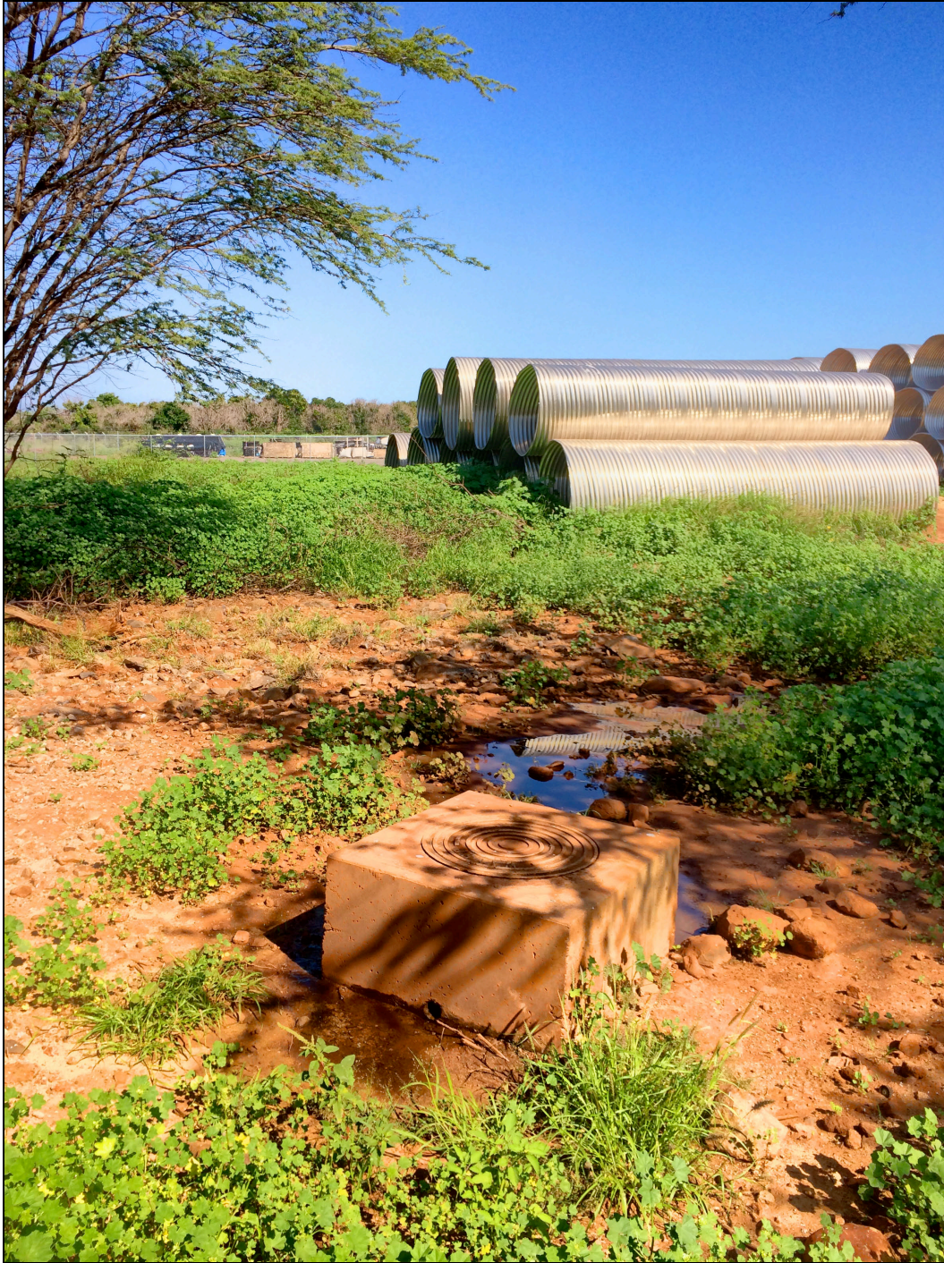
Photo 5: Photo showing the existing waterline manhole near the northeast of the base yard. This water line will be abandoned and a new waterline will be installed along the east and south border of the Piilani Promenade project area.
