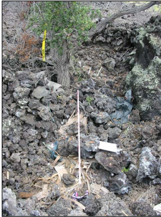
Figure 157. Site -26308, Feature A overview, showing constructed wall in foreground, entrance, and second constructed wall in background, view to east
