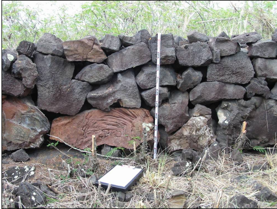
Figure 14. Site -10712, showing wall construction, view to northwest
