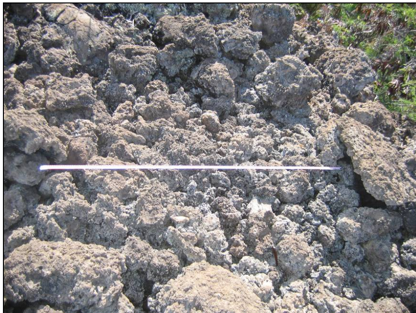
Figure 25. Site -20741, Feature F, paving, view to the southeast
