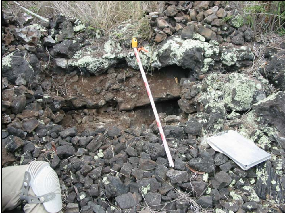
Figure 102. Site -26292, paved surface after excavation
