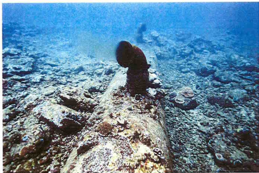
FIGURE 24. Two views of ocean diffuser in Hilo Bay from Hilo Wastewater Treatment Plant. Note abundant coral growth on diffuser pipe and ports that are exposed to effluent plume.
