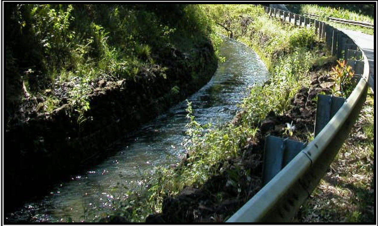
East Maui Irrigation Ditch.
