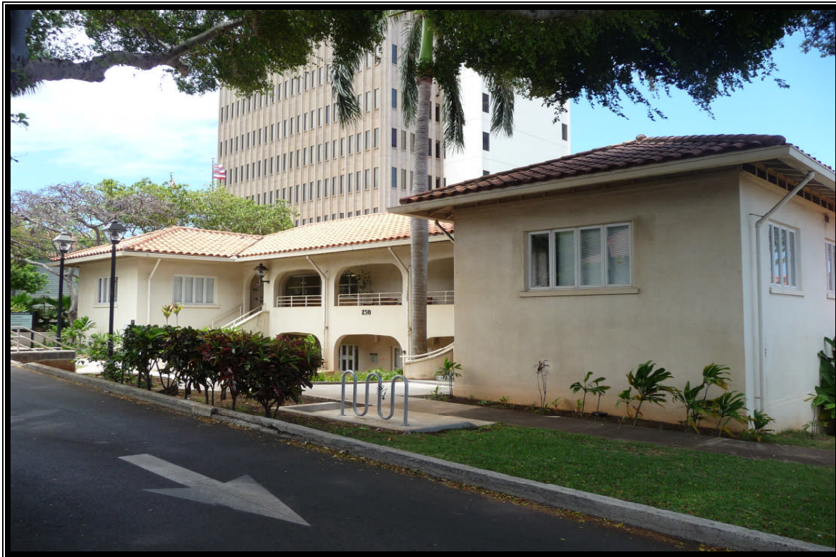
The renovated Kalana Pāku 'i Building, Wailuku.
