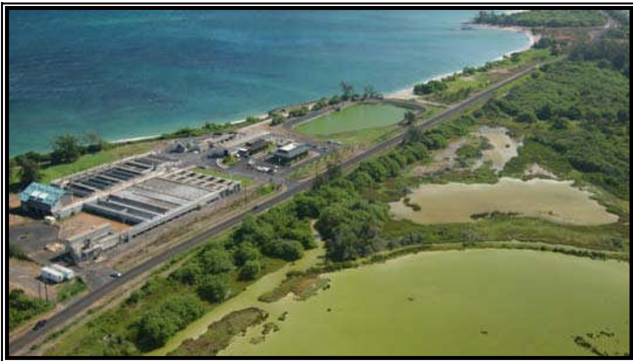
Central Maui Wastewater Reclamation Facility, Kanahā.
