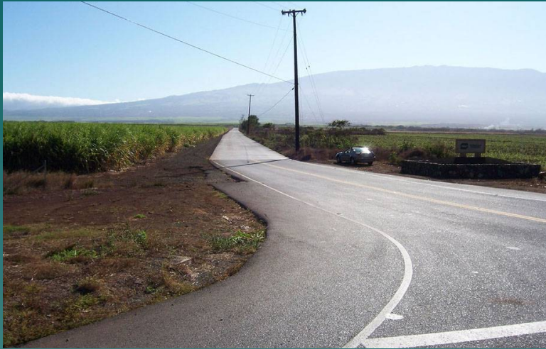
View from the intersection of Mokulele Hwy & Kama`aina Rd (camera facing east)
