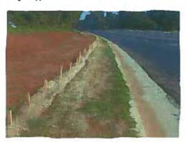
SedimentSTOP consists of a 70% straw / 30% coconut fiber matrix reinforced with a 100% biodegradable netting that is rolled from edge to edge to create a seamless temporary, water-permeable three-dimensional sediment filtrations tructure.
