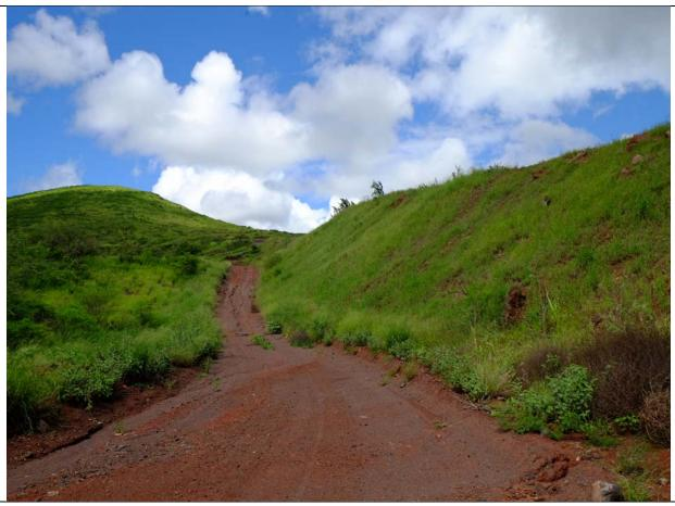
Photo 3, right side, (above), West Road Berm, Hydromulched, without irrigation Photo 4, foreground, (below), West Corner, Hydromulched, without irrigation
