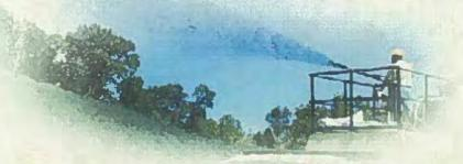
HydraMatriCxna Series high-performance hydraulic erosion control products are made with a proprietary blend of straw, reclaimed cotton plant material, tacklifiers, and polymers.
