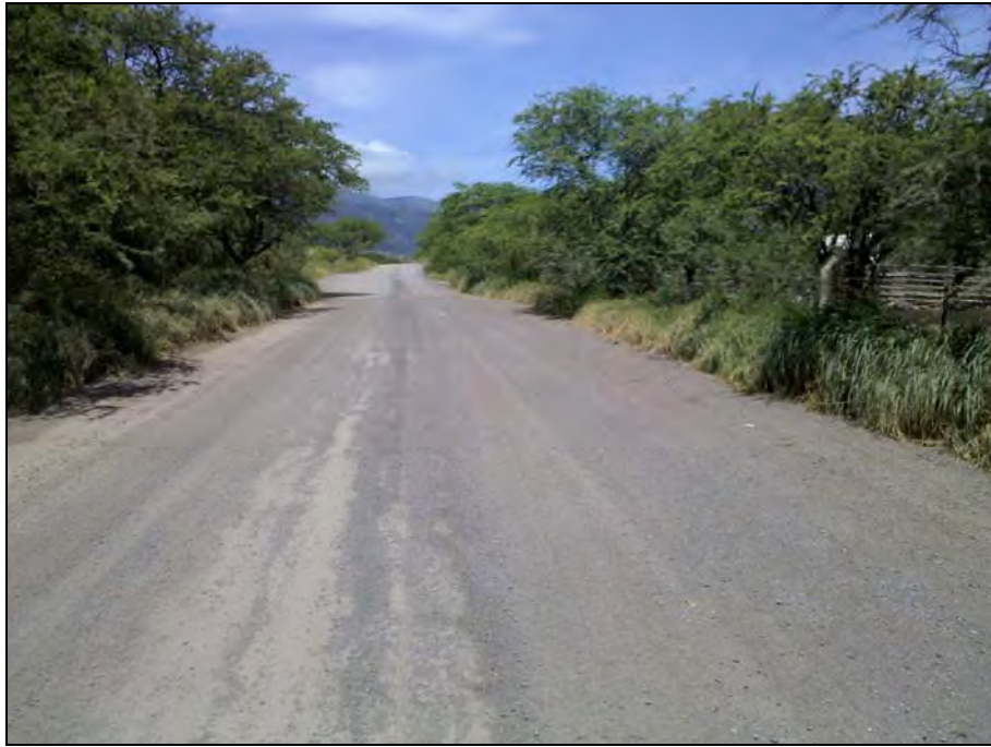
Photo # 4: Graded Access Road Bisecting the Western Portion of the Project Area, View to Northwest.
