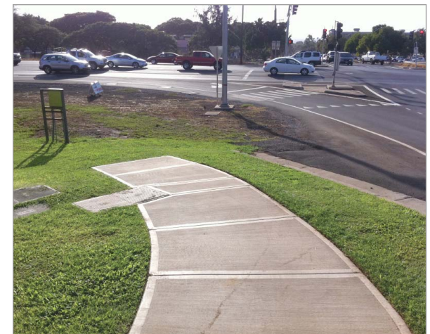
Pedestrian routes are often unconsidered, discontinuous, and unsafe, like this one at the intersection of Lipoa Parkway and Pi'ilani Highway.
