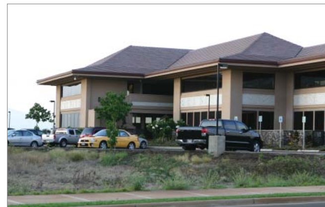
Park Plaza Building in MRTP
